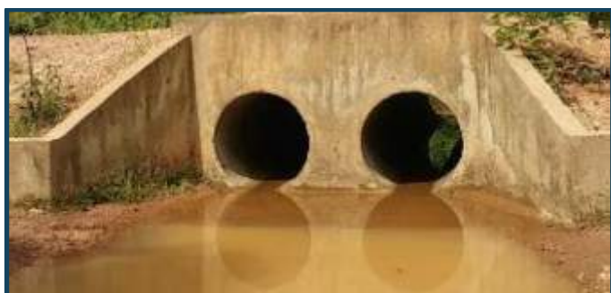
Figure 9.10 Pipe Culvert with Two Barrels
