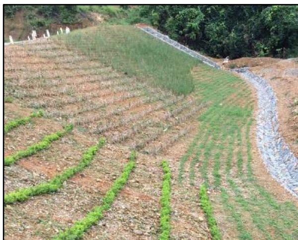
a. Combined shrub line, fascine and grass protection combined with stone and gabion drainage.
