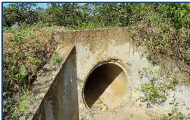
Figure 9.9 Typical Single Barrel Pipe Culvert
