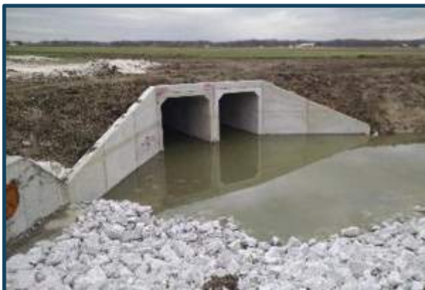
Figure 9.8 Box Culvert with Two Cells
