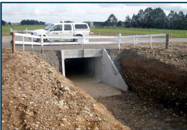
Figure 9.7 Typical Single Cell Box Culvert
