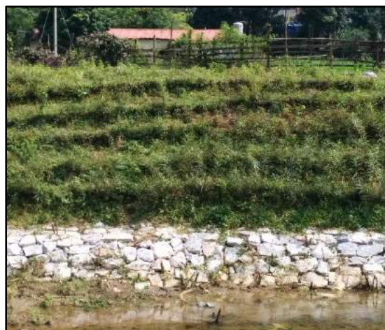
b. Combined rip-rap and brush vegetation protection of roadside river embankment.
