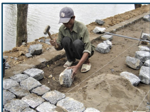
Labour-based construction of cobble road Photo J Cook
