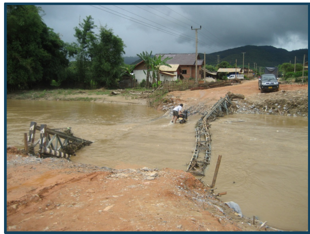
Temporary diversion bridge destroyed by tropical storm floods, Laos PDR
