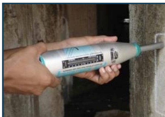
Schmidt Hammer testing
