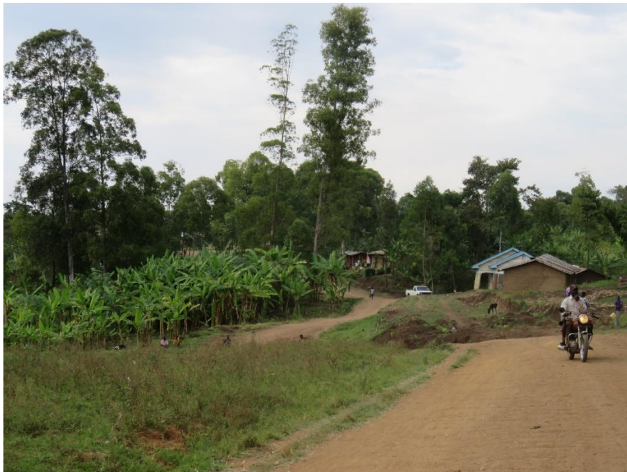
Figure 6 - Horizontal displacement to this originally straight section of road with rotation and structural damage to adjacent buildings
