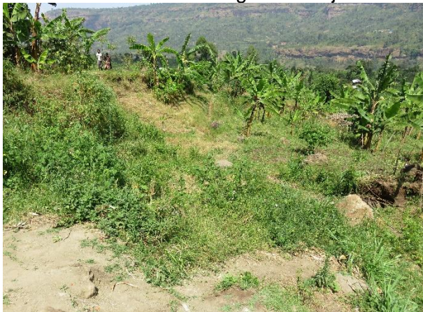
5C Slide scar of earth flow that blocked road
