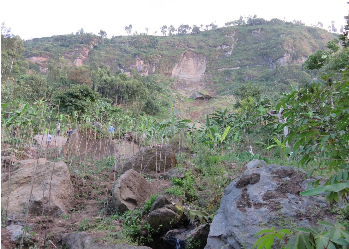
Figure 4 - Rock fall debris in foreground from slide scar in centre of background (Oct 2018)
