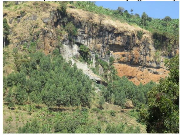
5D Rock falls from natural cliffs above road
