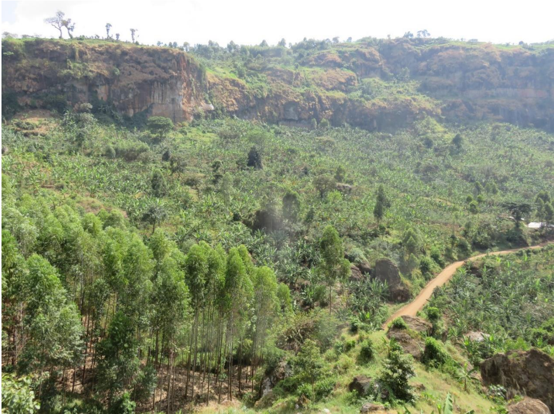
Figure 2 - Cliffs and debris slopes formed in lava and pyroclastic materials, Mount Elgon, where rock falls and toe-slope landslides are common.
