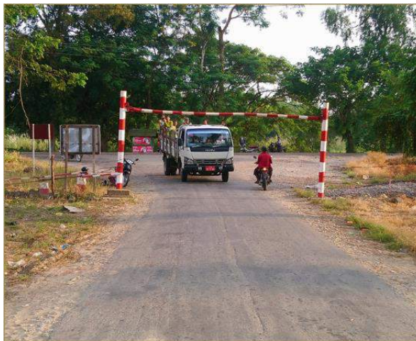
Figure 14-10: Steel gantry to prevent heavy vehicles from entering access roads
