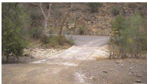
Figure 8-10: A simple stream drift
