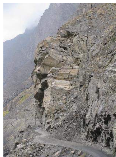
Figure 5-7: Unstable rock mass, cut too steeply with blast damage
