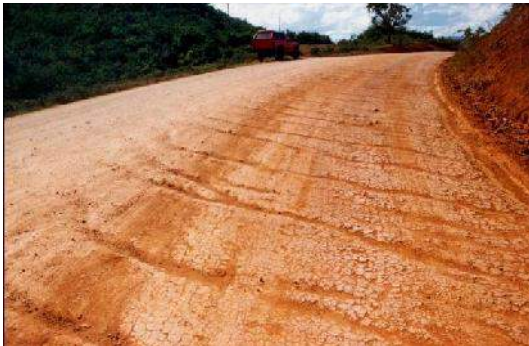
Transverse erosion in fine material
