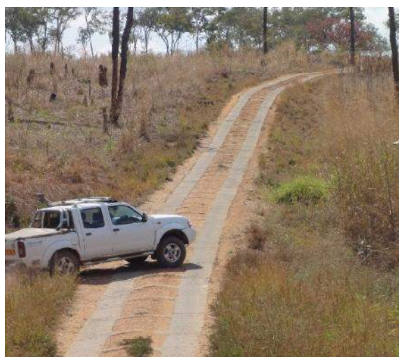
Figure 10-12: Concrete strips to provide access up a steep, sandy section
