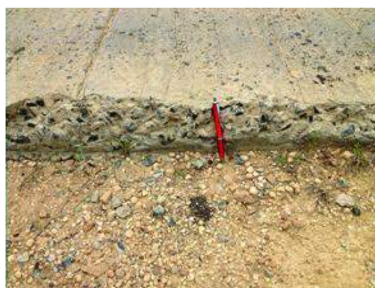
Figure 12-10: Concrete strip road with dangerous edge drop
