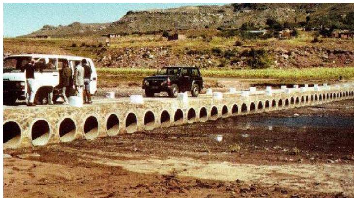
Figure 8-14: A typical Vented drift/Causeway
