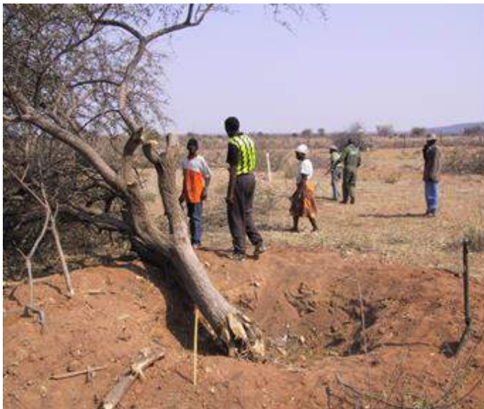
Figure 14-4: Tree removal and de-stumping
