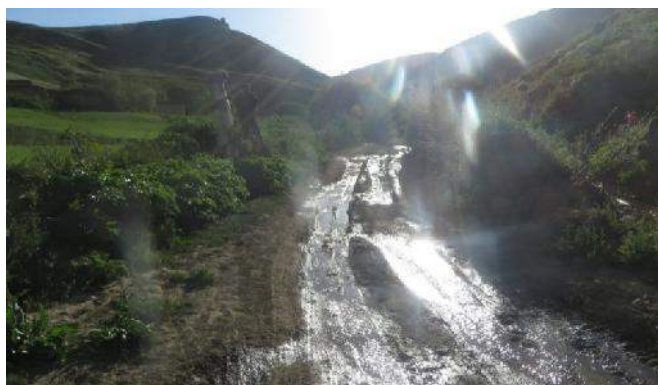
Figure 4-19: Typical road condition in a wet/marshy area
