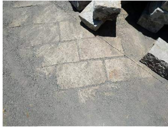
Dressed stone surfacing
