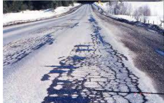
Figure 10-17: Freeze-thaw damage
