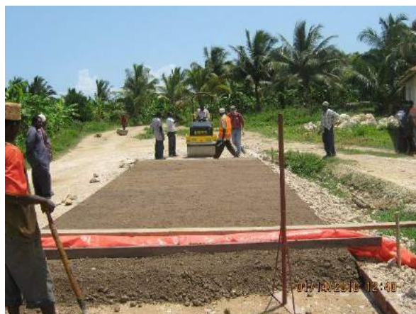
Figure 14-3: Shutter system for construction of ETB base by LBM
