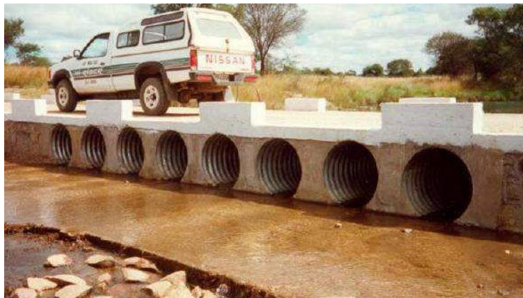
Figure 8-31: Vented drift with apron
