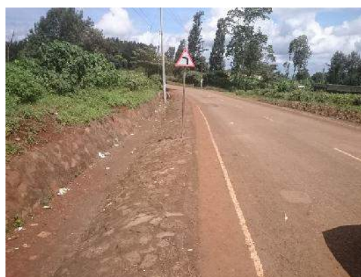
Figure 9-19: Good – Drain lining connected to edge of surfacing
