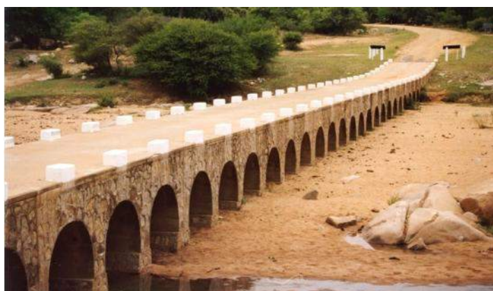
Figure 8-15: Example of submersible bridge
