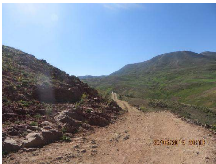
Figure 5-6: Siltstone or fine-grained sandstone exposed in the cut slope
