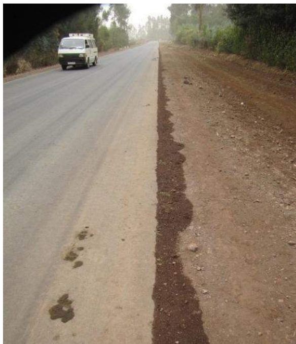
Figure 9-4: Infiltration of water through a permeable surfacing
