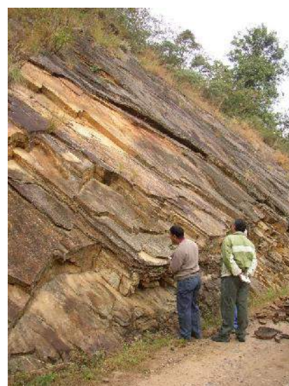
Figure 5-5: Joint-controlled stability in cut slopes
