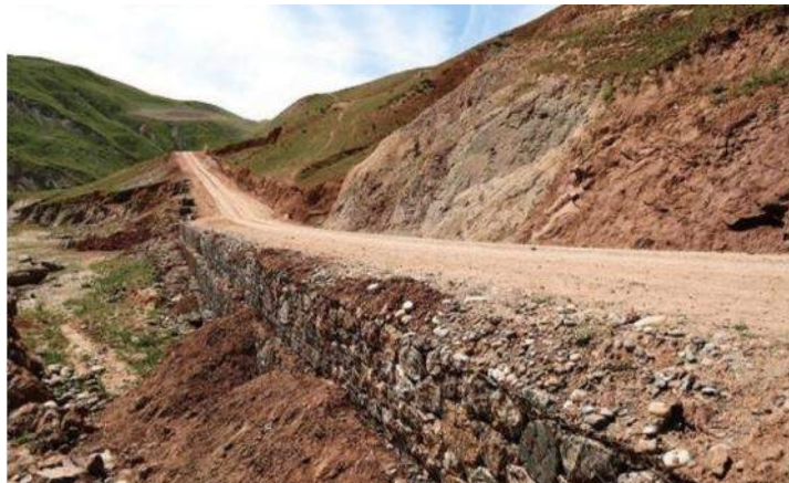
Figure 6-8: Variable deposits of residual soils visible in cut-slopes
