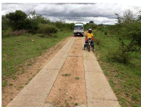
Figure 12-10: Concrete strip road with dangerous edge drop
