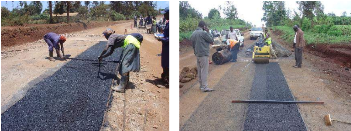
Figure 12-7: Levelling and compaction of CMA
