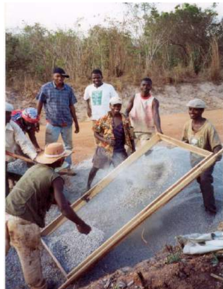
Figure 14-5: Screening of aggregates
