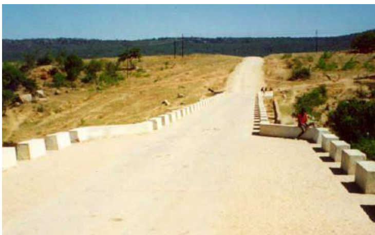
Figure 8-8: Example of a restricted width on water crossing structure
