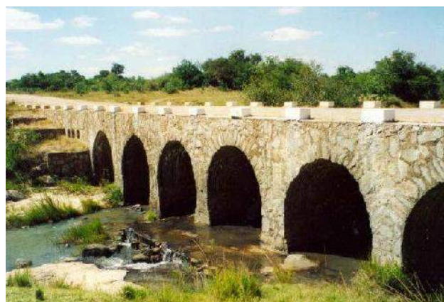
Figure 8-27: Example of a masonry arch culvert
