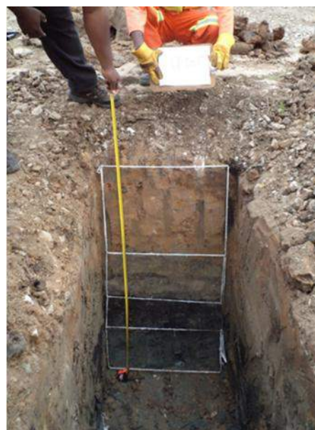
Figure 4-4: Logging of subgrade profile
