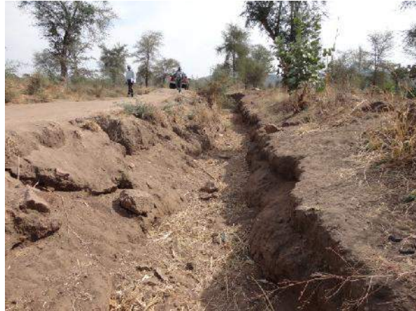
Figure 4-13: Gully formation in erodible soil
