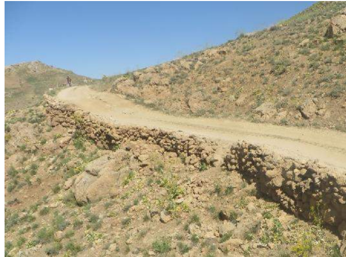
Figure 5-10: Use of locally available materials to support the road edge
