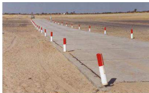
Figure 8-11: A drift crossing a wide floodplain
