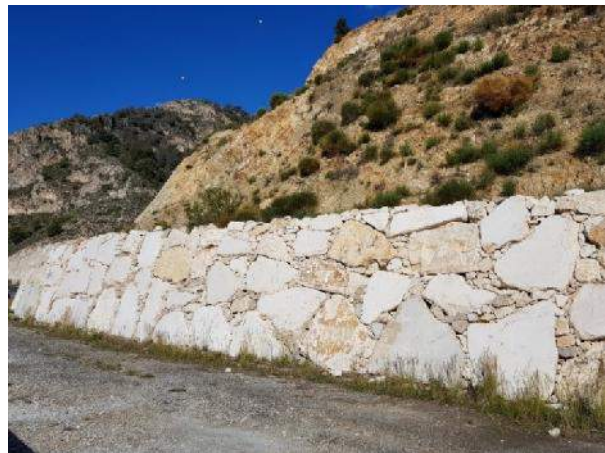
Figure 5-14: Typical retaining and revetment wall constructed of interlocking boulders
