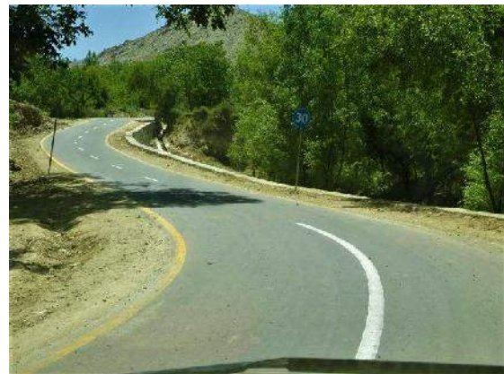
Figure 1-1: Typical LVRR in Afghanistan
