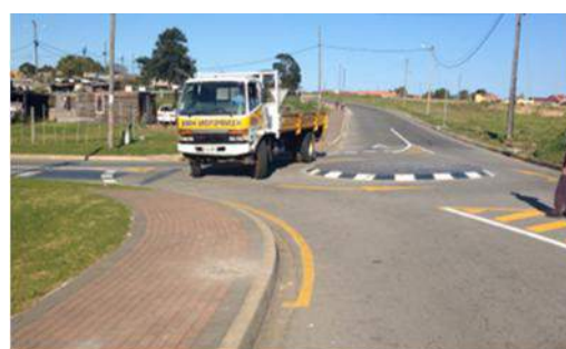
Figure 4-10: Mini circle used as a speed reducing measure in a village
