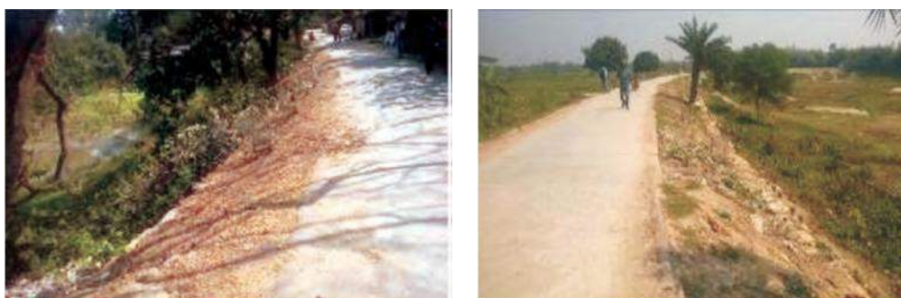
Figure 3-5: Limited maneuvering and recovering space on embankments
