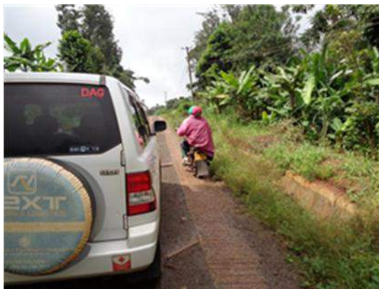
Figure 3-4: Typical problems encountered on rural roads
