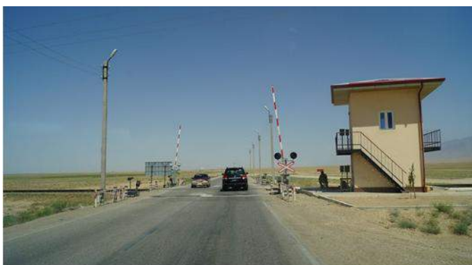
Figure 4-23: : Typical rail level crossing on a road in northern Afghanistan
