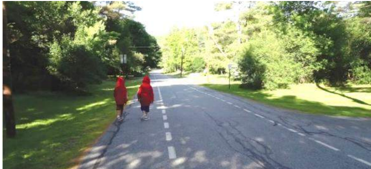
Figure 4-18: Example of road marking on rural LVR
