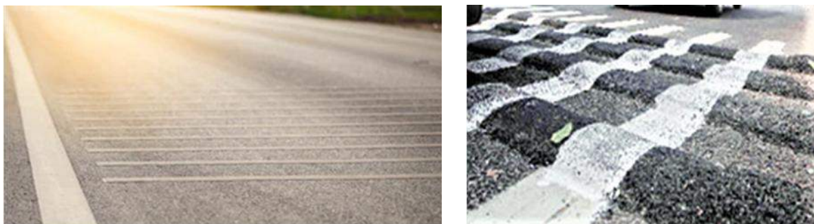
Figure 4-5: Examples of well designed (left) and poorly designed (right) rumble strips
