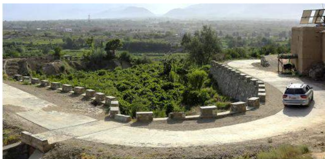
Figure 4-21: Masonry work providing an effective barrier on steep drop-offs
