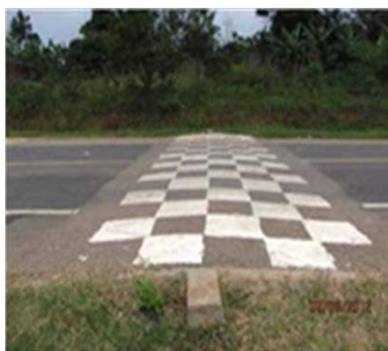
Figure 4-7: Watts speed hump profile
