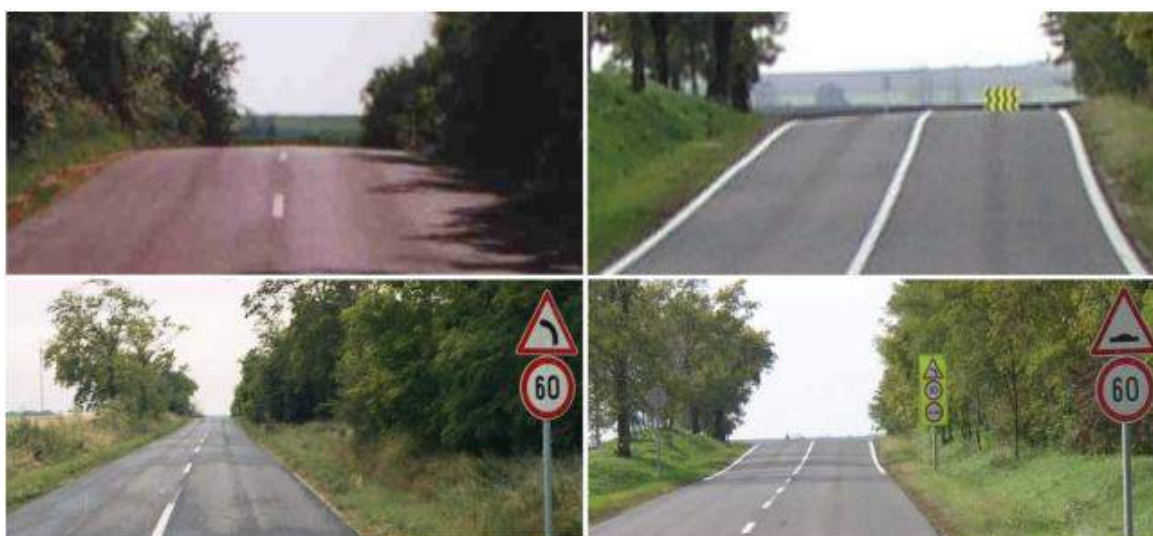
Figure 2-5: Use of edge markings to improve road safety on vertical crest curve
