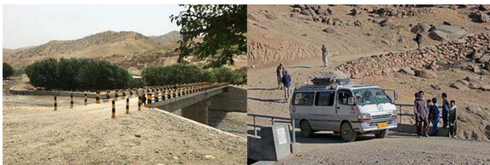
Figure 4-26: Examples of protected bridge approach and bridge railings
