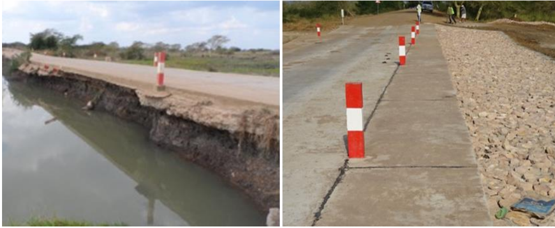
Figure 5 - Example site in Mozambique's Gaza Province, where the road has been adapted to address overtopping-induced erosion
