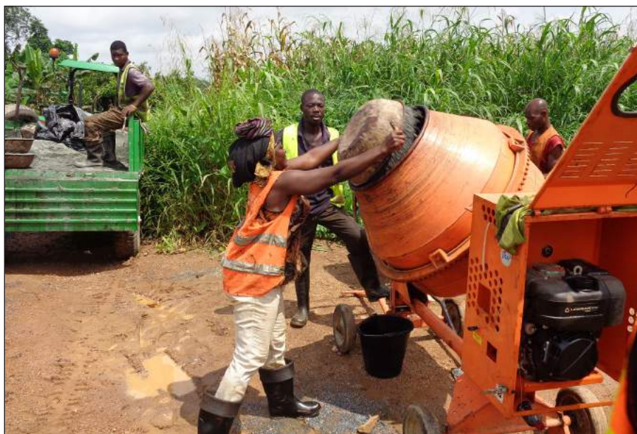
Figure A.3.4: Participation of women in road works on LVRs
