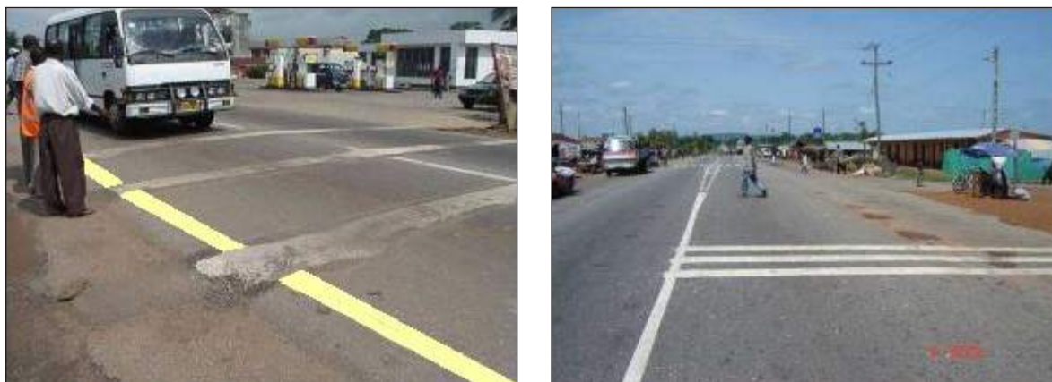
Figure A.7.6: Rumble strip application
