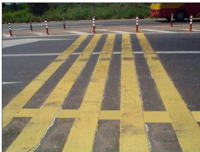
Figure A.7.7: Jiggle bars application
