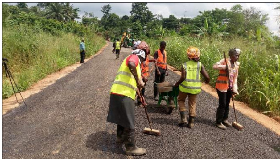
Figure A.3.3: Labor-based technology on an LVR
