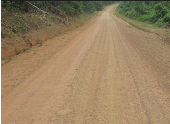
Figure B.8.6: Gravel Road
