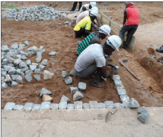
Figure B.9.16: Construction of Cobble Stone Paving
