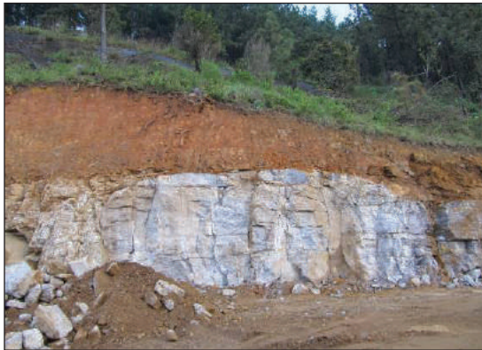
Abrupt interface between WG V and WG I-II, i.e. rock that requires blasting is found directly beneath residual soil.
