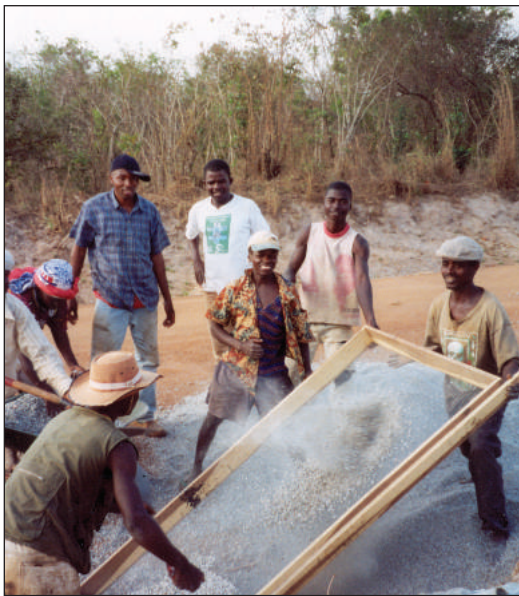
Figure B.9.1: Screening of aggregate for road surfacing
