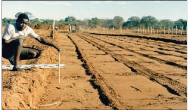
Figure B.4.12: Collapse settlement following impact compaction
