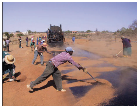
Figure B.9.19: Spreading gravel using LBM
