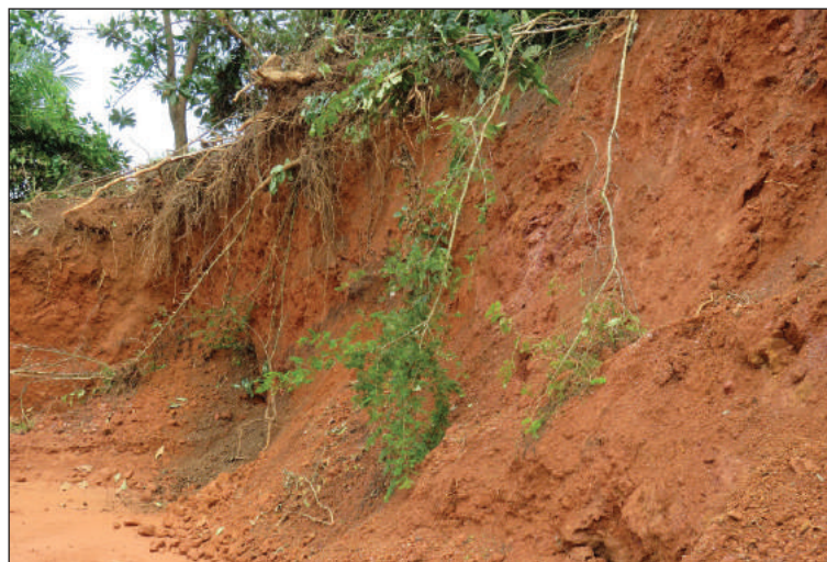
Figure B.10.3: Typical borrow pit excavation face in weathered rock
