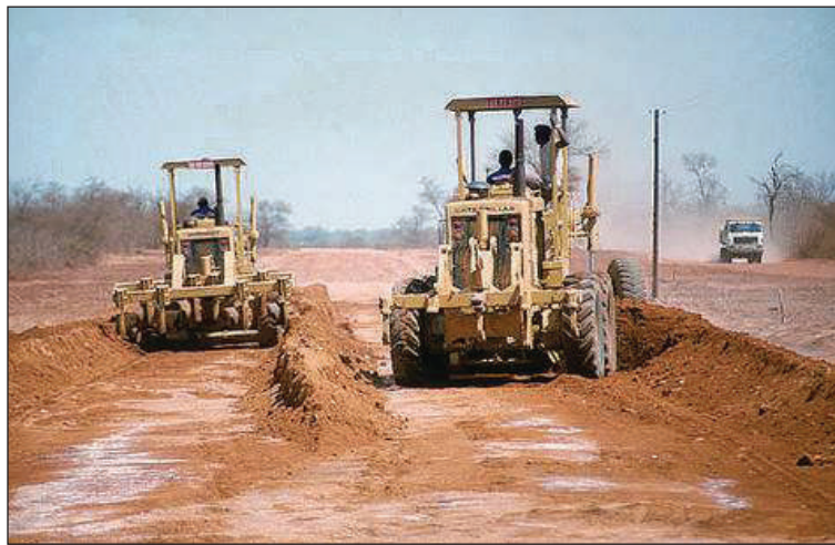
Figure B.9.5: Motor graders processing materials on the road
