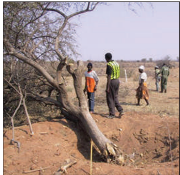
Figure B.9.2: De-stumping of trees
