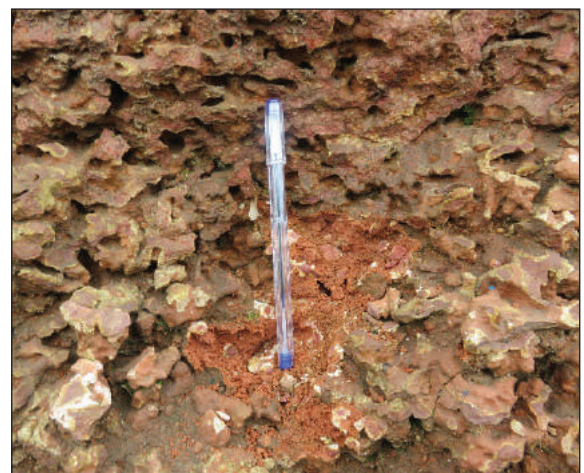
Typical welded lateritic gravel
