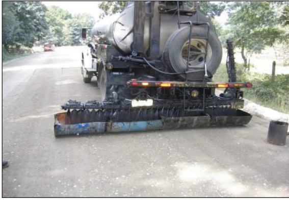
Figure B.9.14: Verifying transverse distribution of binder
