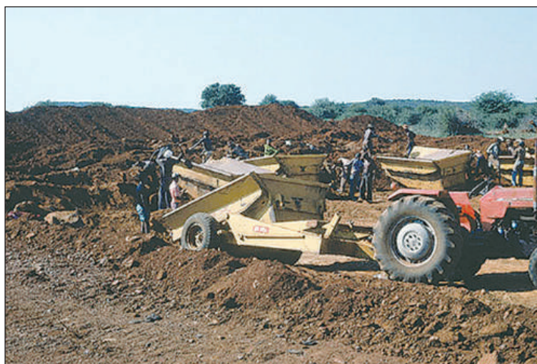
Figure B.9.4: The use of labor and small tractor-drawn trailers
