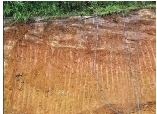
WG II-III overlies WG V due to increased weathering at depth caused by groundwater flow. Creates weaker materials with depth.
