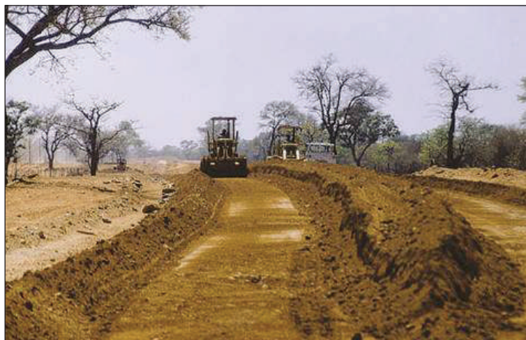
Figure B.9.10: Mixing of materials on the road with a motor grader
