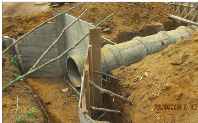
Figure C.6.2: Reinforced concrete pipe culvert
