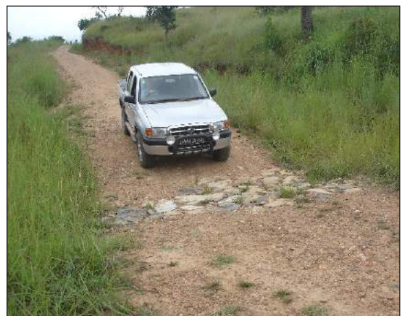
Figure C.4.14: Simple drift using hand packed stone
