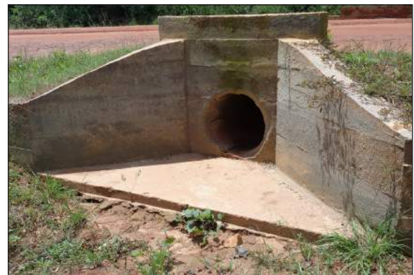
Figure C.6.5: Concrete apron at culvert outlet
