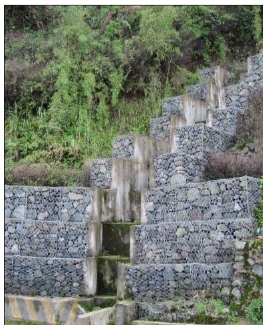
Figure C.6.11: Gabion cascade
