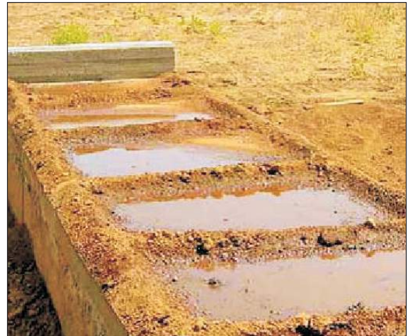
Figure C.8.7: Curing concrete slab by ponding
