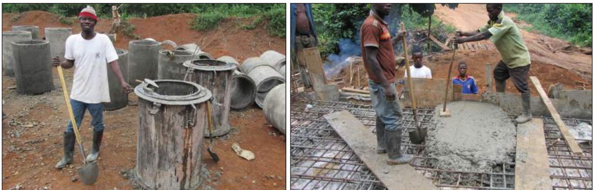
Figure C.8.13: Concrete culvert ring production Figure C.8.14: Constructing reinforced concrete slab
