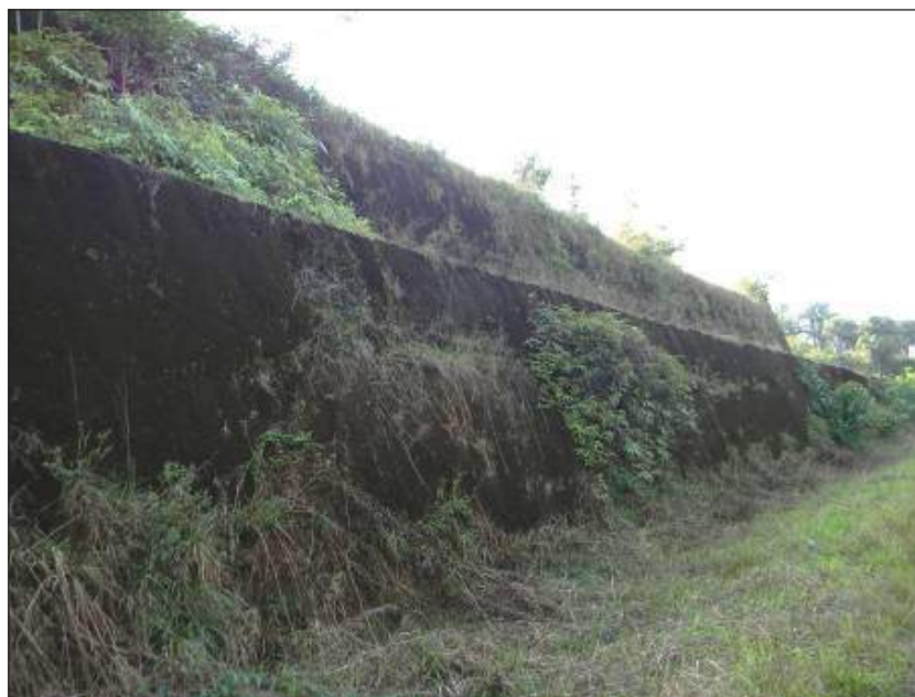
Figure C.7.9: Benched cut slope in residual soils
