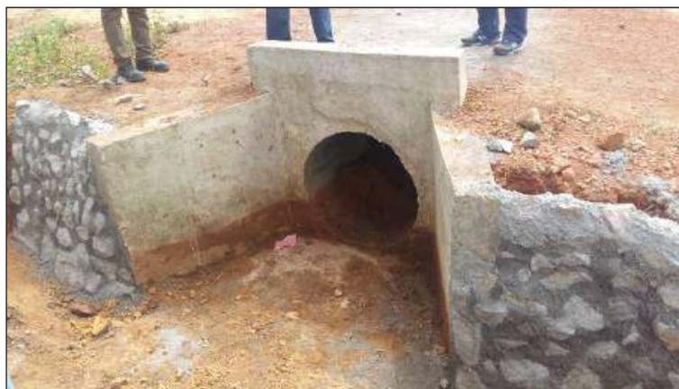
Figure C.8.15: Stone pitched embankment slopes behind wingwalls
