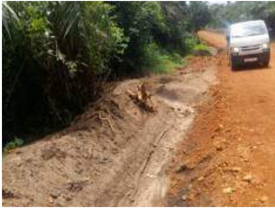
Figure C.4.4: Turn-out on an LVR
