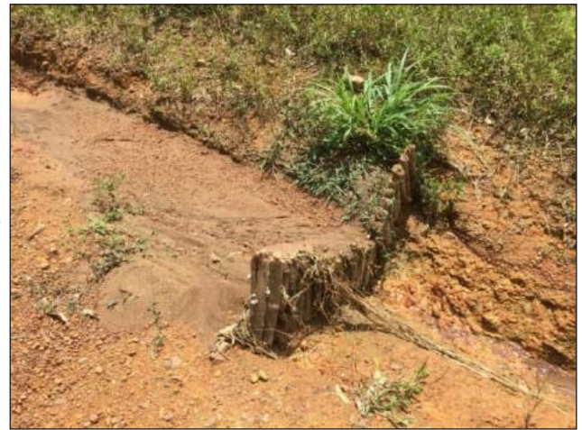
Figure C.6.14: Scour check made from wooden stakes
