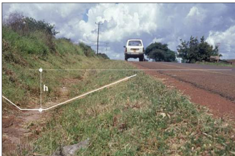
Figure C.2.1: A well-drained pavement
