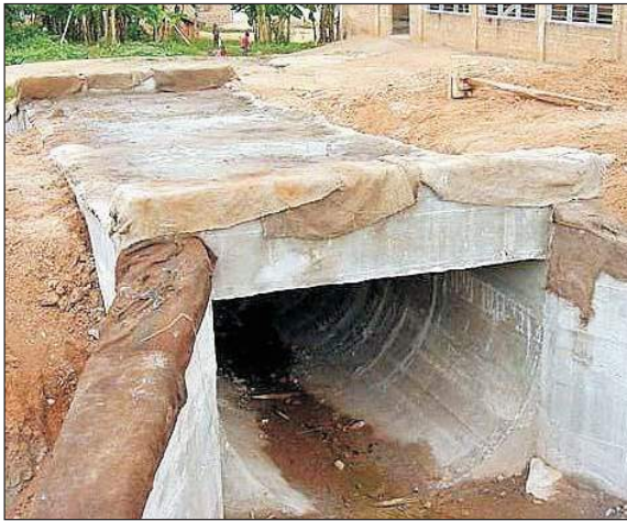
Figure C.8.6: Curing of concrete with wet hessian sacking
