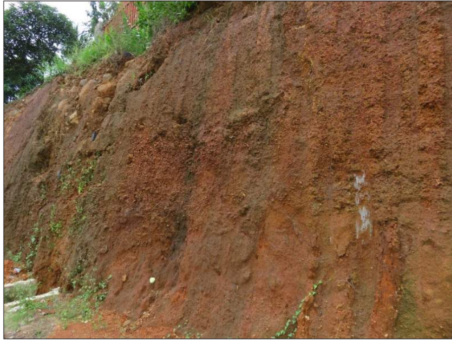
Figure C.7.8: Welded laterite gravels standing steeply in roadside cut slope
