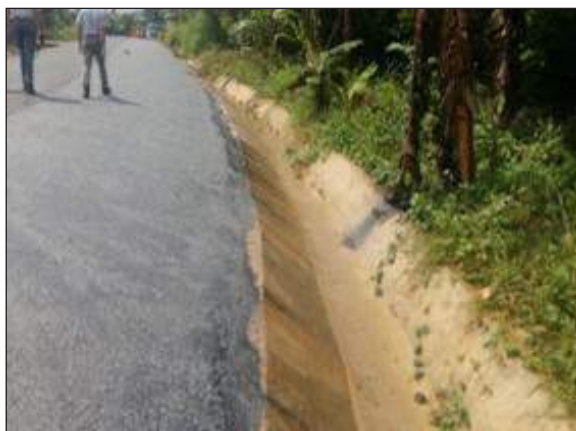
Figure C.4.2: Concrete lined trapezoidal drain
