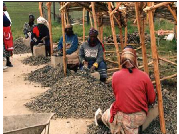
Figure C.8.3: Aggregate being crushed by hand
