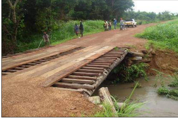
Figure C.8.19: Timber bridge deck
