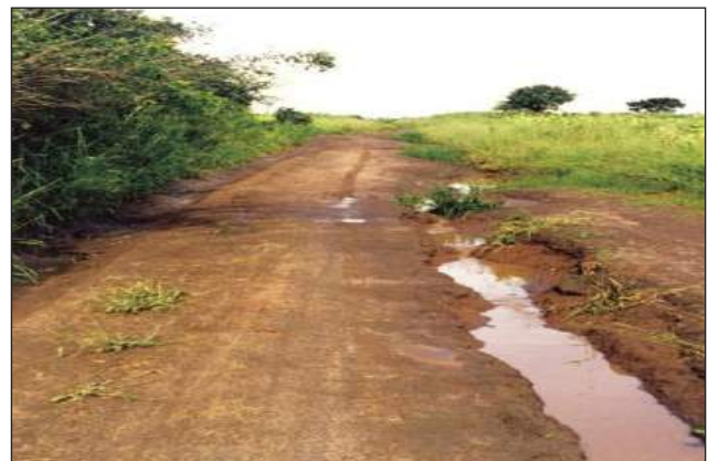
Figure C.4.15: Poor drainage on flat ground
