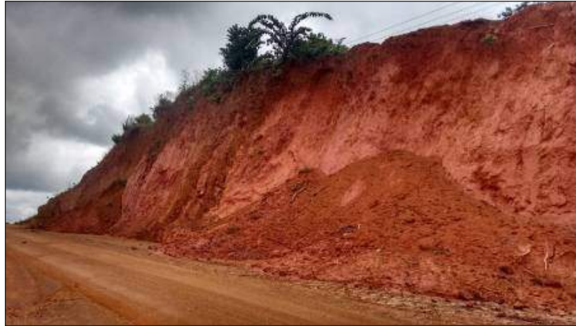
Figure C.7.3: Failure of the upper portion of the cut slope in the weathered mantle
