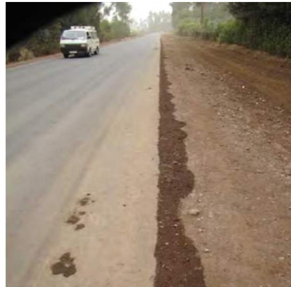
Figure C.2.4: Infiltration of water through a permeable surfacing
