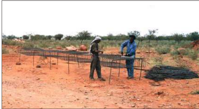
Figure C.8.4: Steel reinforcement cage being assembled
