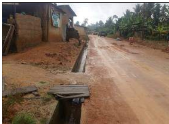
Figure C.4.3 Concrete lined U-drain
