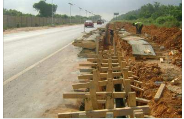
Figure C.8.20: Timber formwork
