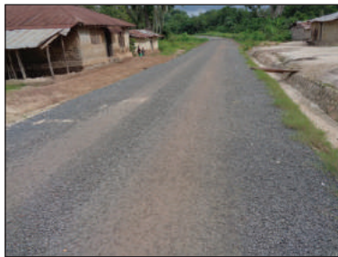
Surface dressing (chip seal)
