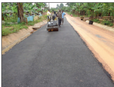
Cold Mix Asphalt
