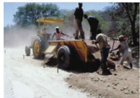
Off-loading and spreading gravel by labor-based methods
