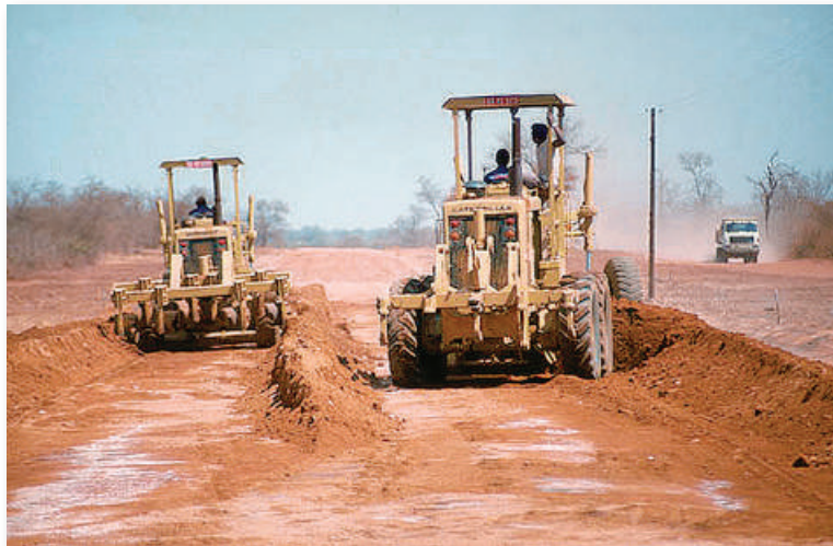
Figure B.9.5 Motor graders are versatile for processing materials on the road
