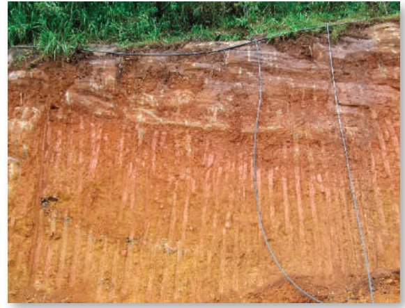
WG II-III overlies WG V due to increased weathering at depth caused by groundwater flow. Creates weaker materials with depth
