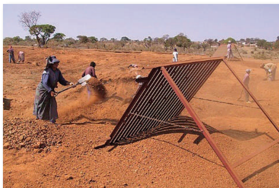
Figure B.9.16 Screening aggregate by LBM
