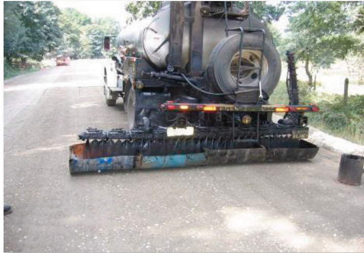
Figure B.9.14 Verifying transverse distribution of binder
