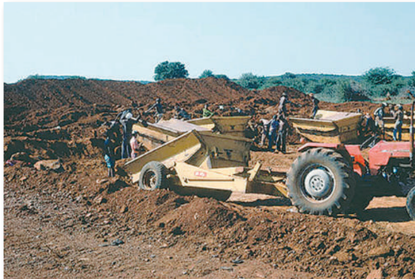
Figure B.9.4 The use of labourers and small tractor-drawn trailers
