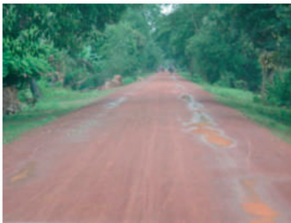
Figure B.8.6 Gravel road
