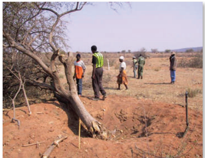
Figure B.9.2 De-stumping of trees
