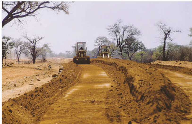
Figure B.9.10 Mixing of materials on road with a motor grader
