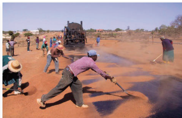
Figure B.9.17 Spreading gravel using LBM
