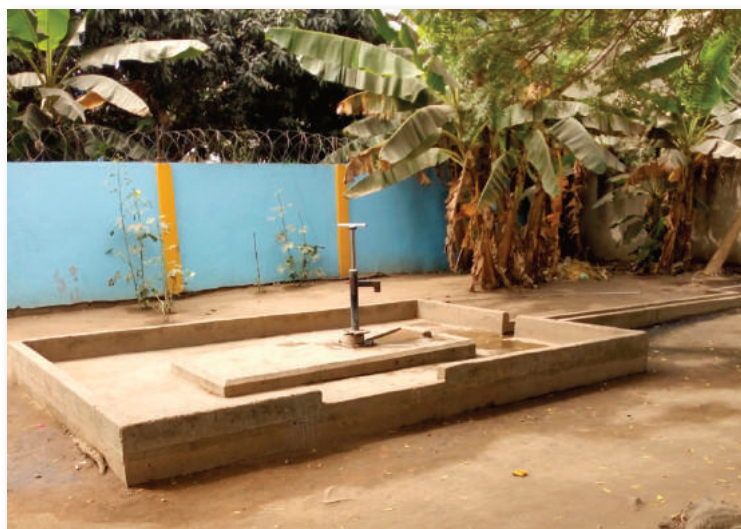
Figure A.3.1 Installation of water pump as a Complementary Intervention
