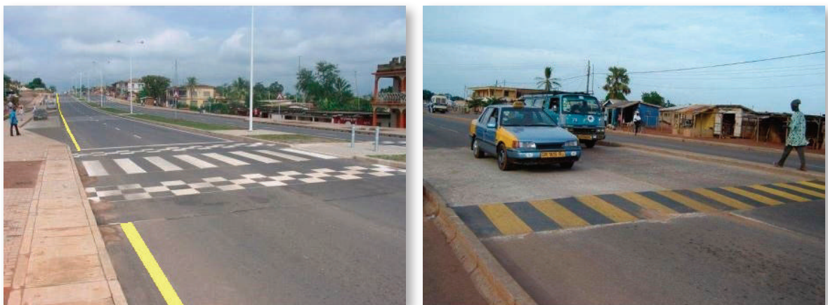
Figure A.7.1 Speed humps
