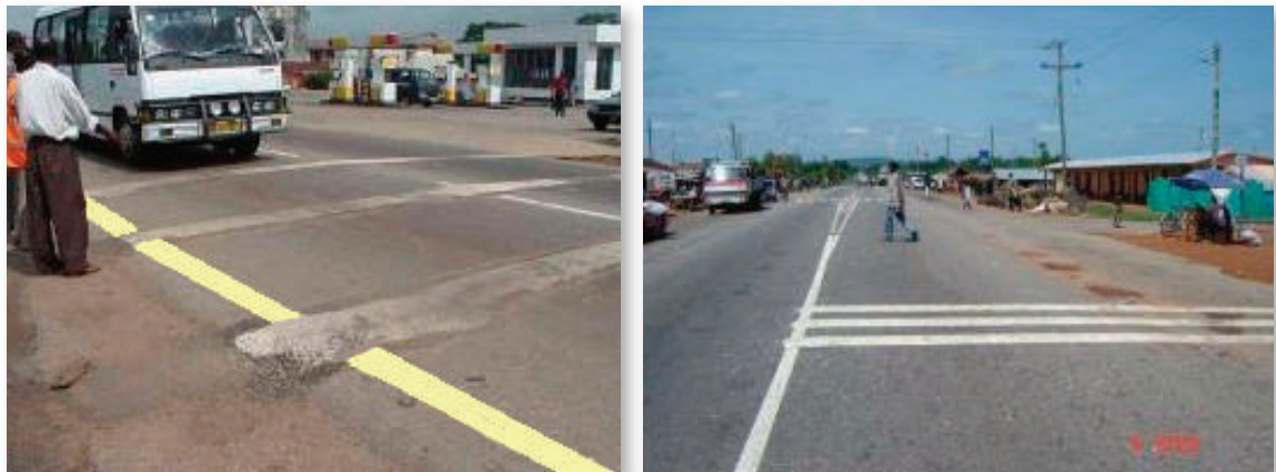
Figure A.7.6 Rumble strips
