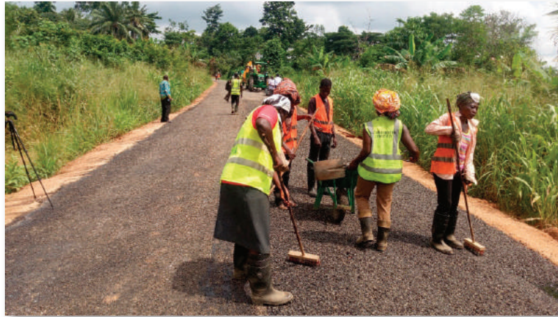
Figure A.3.3 Labour-based technology on a Low Volume Road
