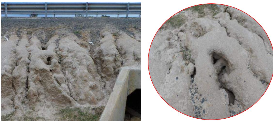
Figure 4-13: Piping in dispersive soils
