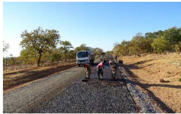
Figure 1-1: Construction of a LVR in Malawi
