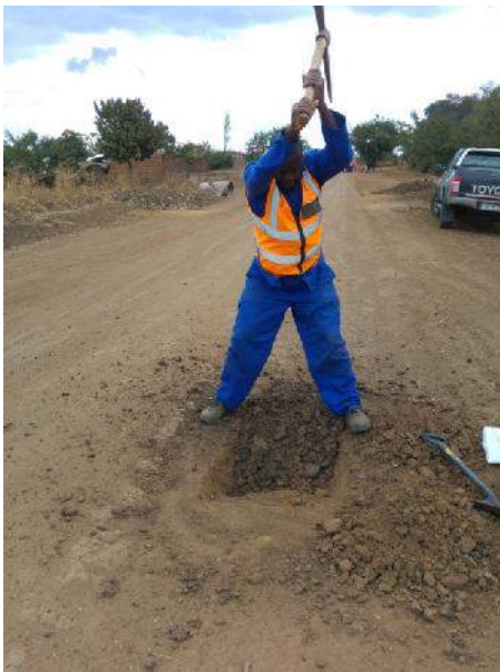
Figure 4-4: Excavation of test pit by labour
