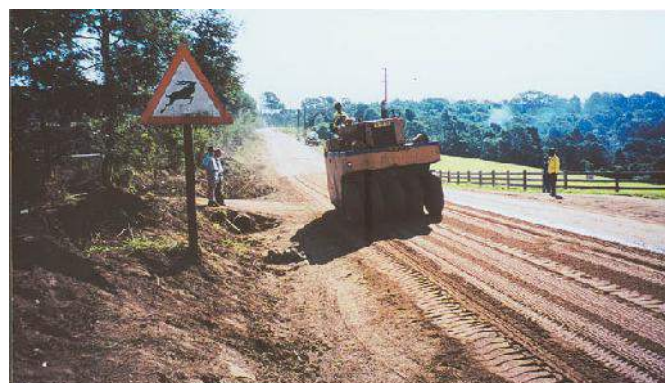
Figure 11-6: Extensive rolling of an Otta Seal is essential to achieve a good result
