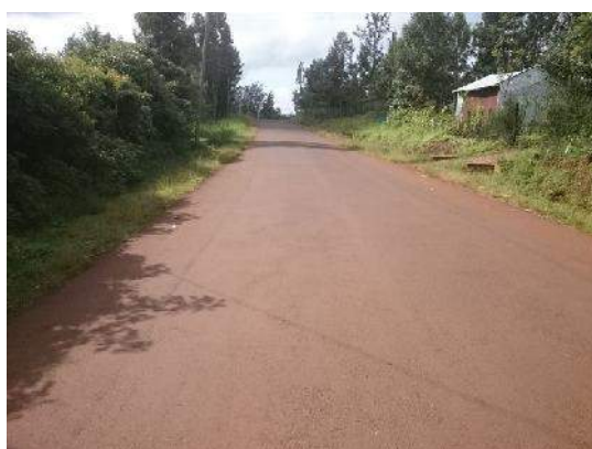
Figure 13-3: LVS base and CMA surfacing constructed by LBM
