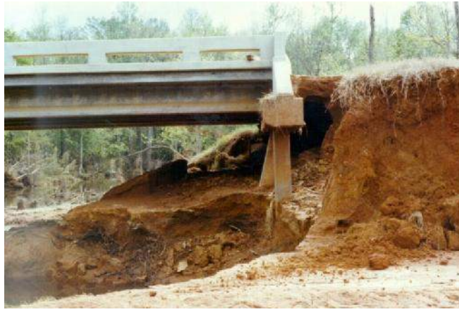
Figure 4-26: Typical bridge scour
