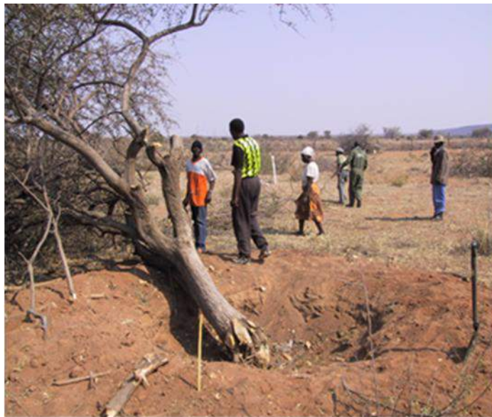
Figure 13-5: Tree removal and de-stumping
