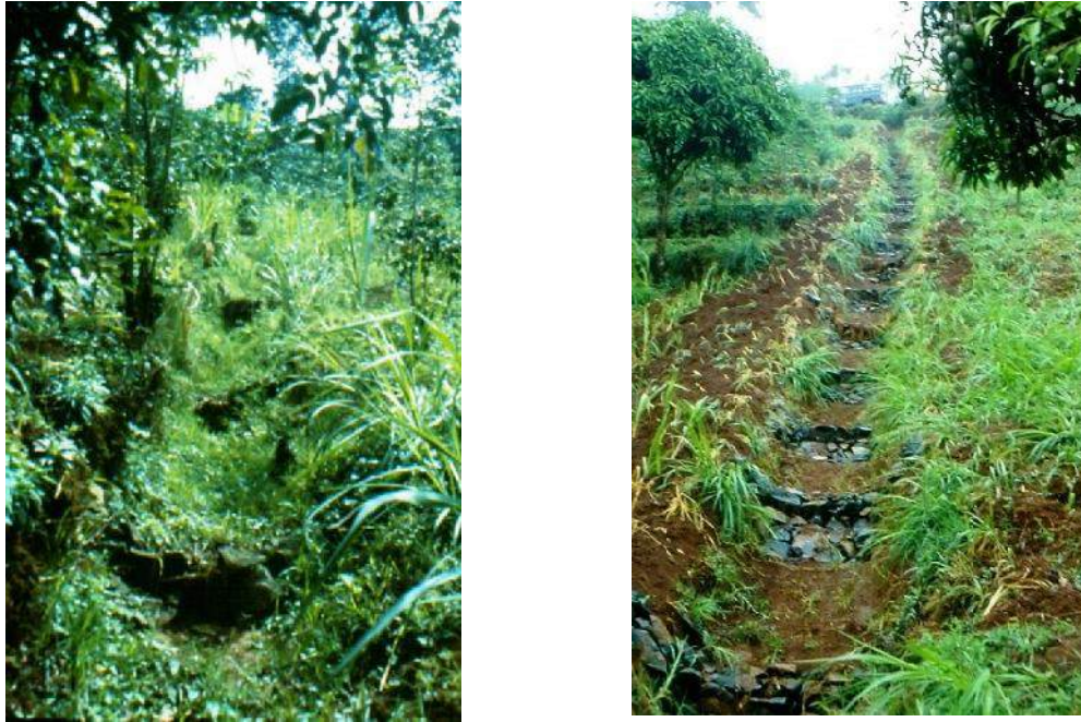
Figure 8-20: Grassed waterways with and without checkdams
