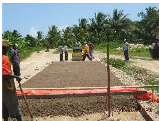
Figure 13-4: Shutter system for construction of ETB base by LBM
