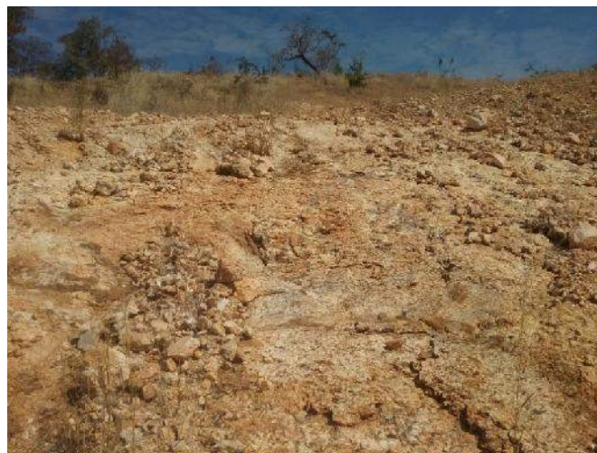
Figure 5-1: Variable weathering in borrow source
