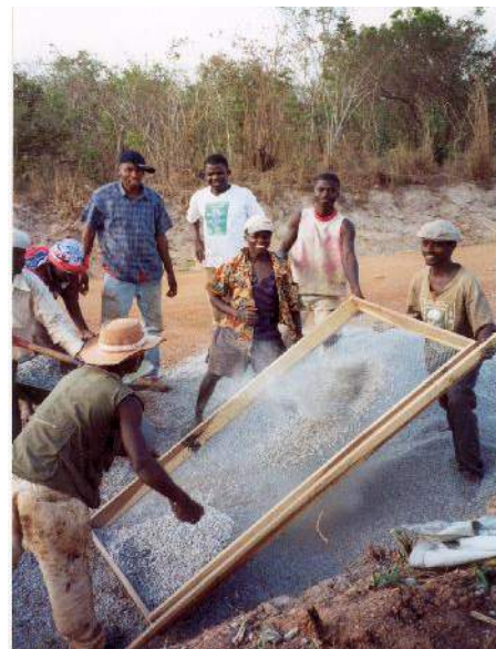
Figure 13-6: Screening of aggregates
