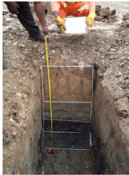
Figure 4-5: Logging of subgrade layers
