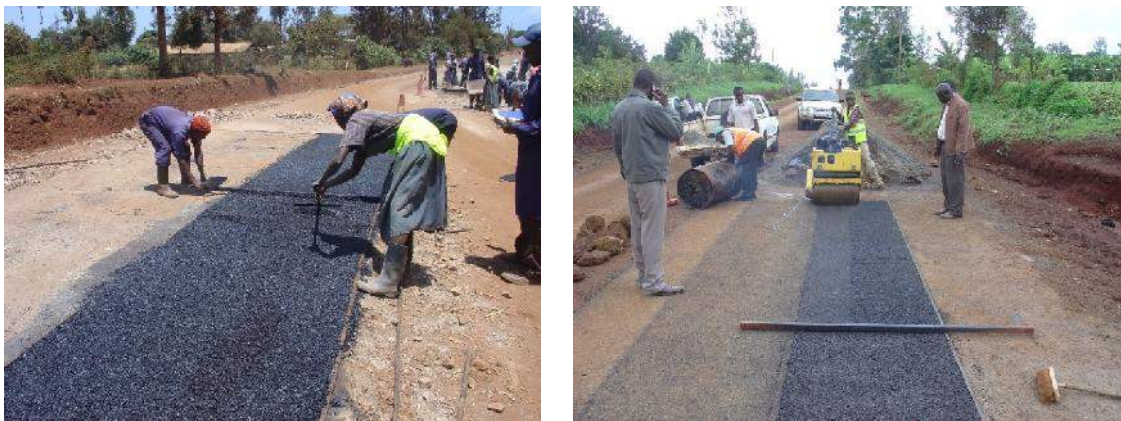
Figure 11-7: Levelling and compaction of CMA
