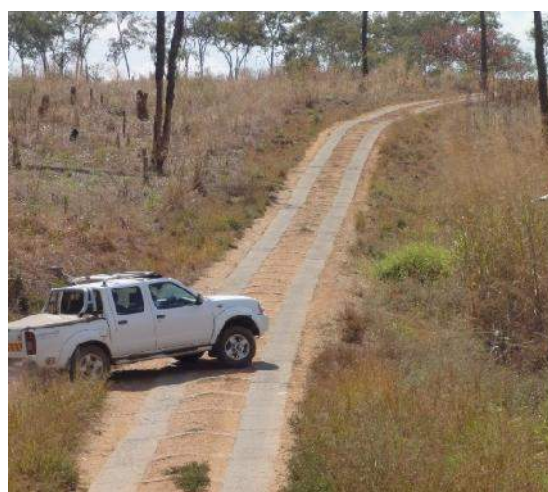
Figure 9-15: Concrete strips to provide access up a steep, sandy section
