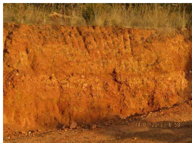
Figure 5-3: Typical laterite borrow pit showing variable nature of the material
