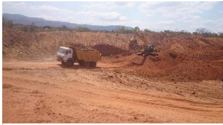
Figure 4-22: Sufficient construction material of the required quality must be located
