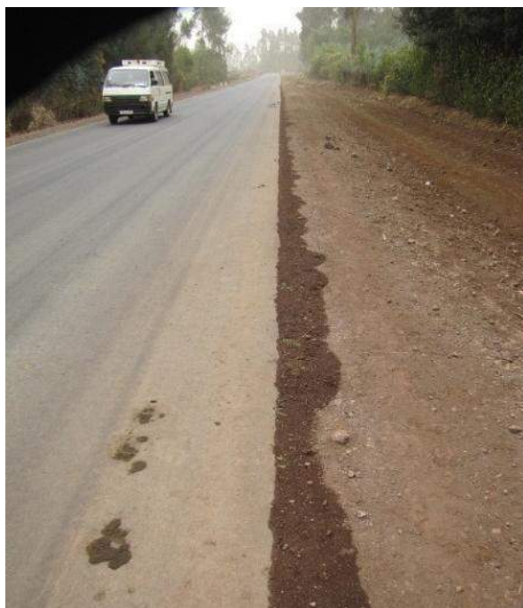
Figure 8-4: Infiltration of water through a permeable surfacing
