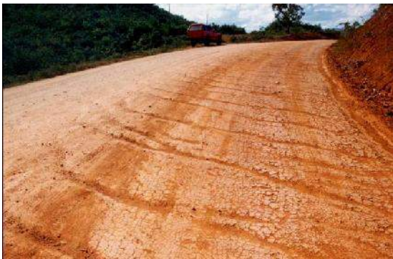
Transverse erosion in fine material
