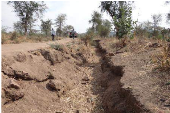
Figure 4-14: Gully formation in erodible soil (Ntcheu District, Central Region)
