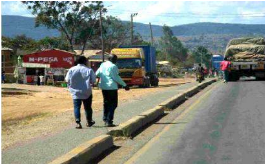
Segregated shoulder using barrier kerb
