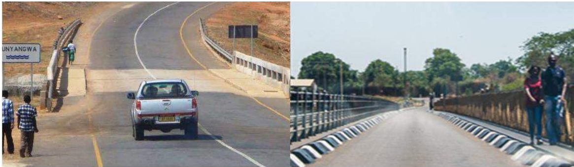
Figure 4-22: Bridges with separate walkway
