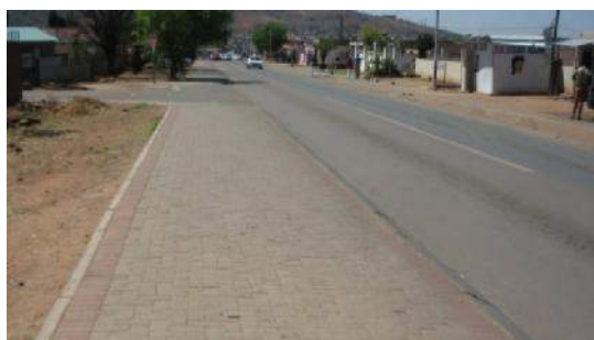
Figure 6-4: Wider than normal sidewalk
