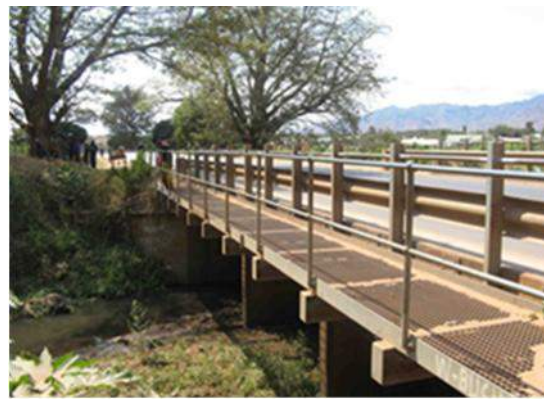
Segregated footpath on narrow bridge
