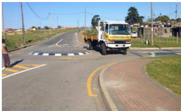
Figure 4-8: Mini circle intersection used as a speed reducing measure on the through-road
