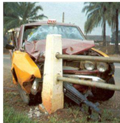
Badly designed bridge railing
