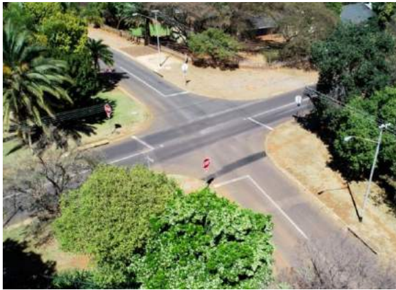
Figure 8-10: Four-way stop between two class 4 Streets
