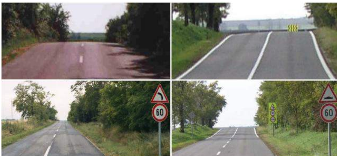
Figure 2-6: Use of edge markings to improve road safety on vertical crest curve
