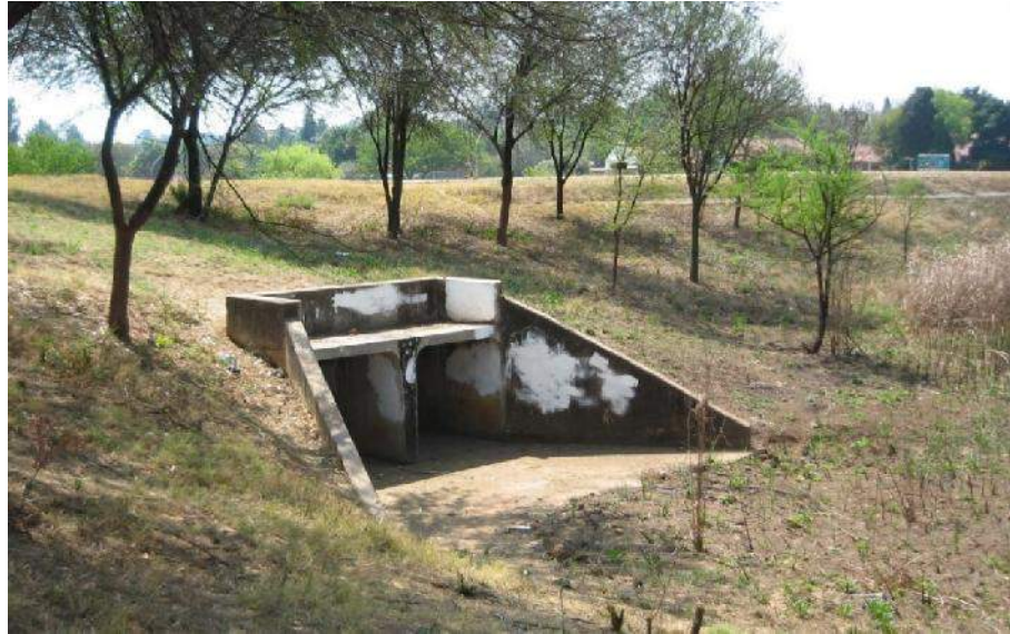
Figure 5-1: Attenuation dam and inlet to outlet structure
