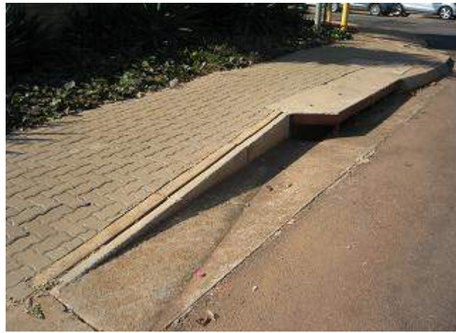
Figure 5-4: Kerb inlet
