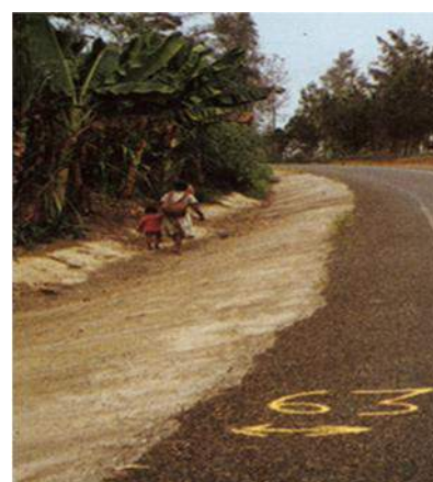
Well designed side drain
