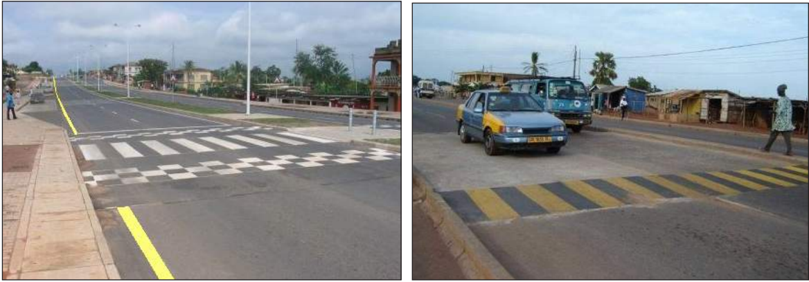
Figure A.7.1: Speed hump application
