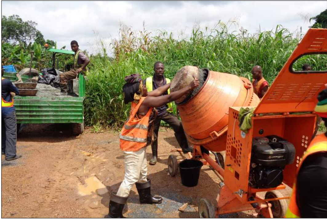
Figure A.3.4: Participation of women in road works on LVR
