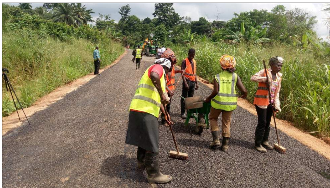
Figure A.3.3: Labour-based technology on a LVR
