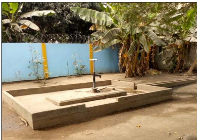
Figure A.3.1: Installation of a water pump as a Complementary Intervention
