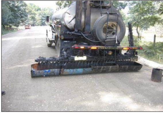
Figure B.9.14: Verifying transverse distribution of binder
