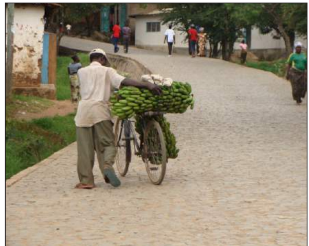
Figure B.9.17: Cobble Stone Paving
