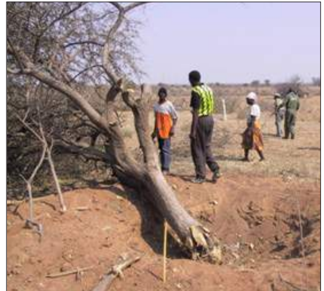
Figure B.9.2: De-stumping of trees
