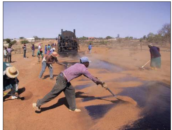
Figure B.9.19: Spreading gravel using LBM
