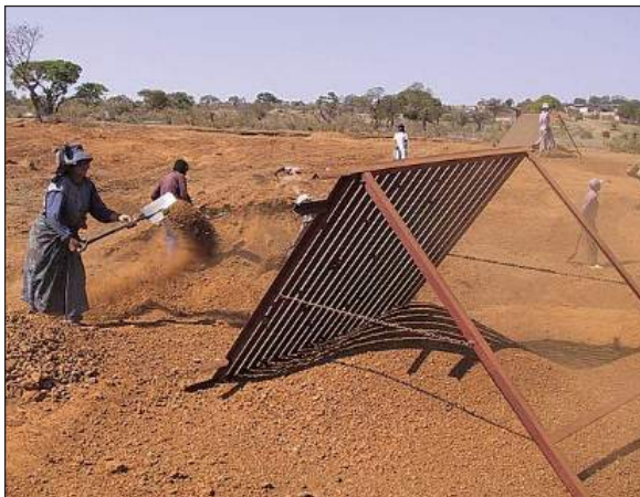
Figure B.9.18: Screening aggregate by LBM
