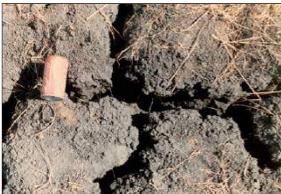
Figure B.4.6: Expansive soil exhibiting wide shrinkage cracks
