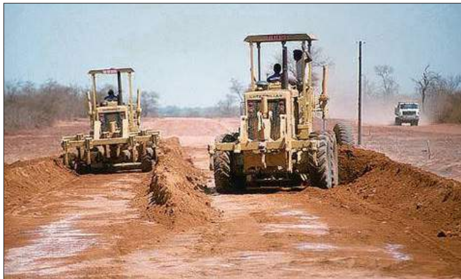
Figure B.9.5: Motor graders are versatile for processing materials on the road
