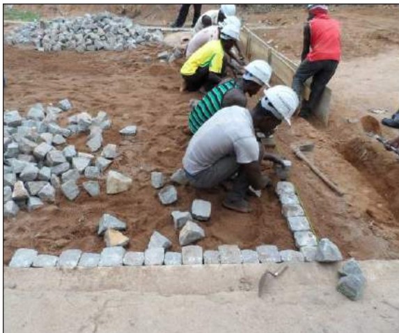
Figure B.9.16: Construction of Cobble Stone Paving
