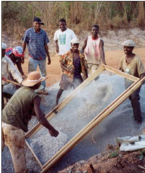
Figure B.9.1: Screening of aggregate for road surfacing
