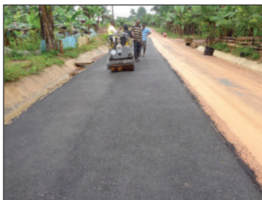
Cold Mix Asphalt
