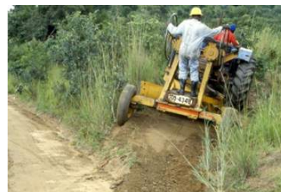
The towed grader can be used to clean turn out drains
