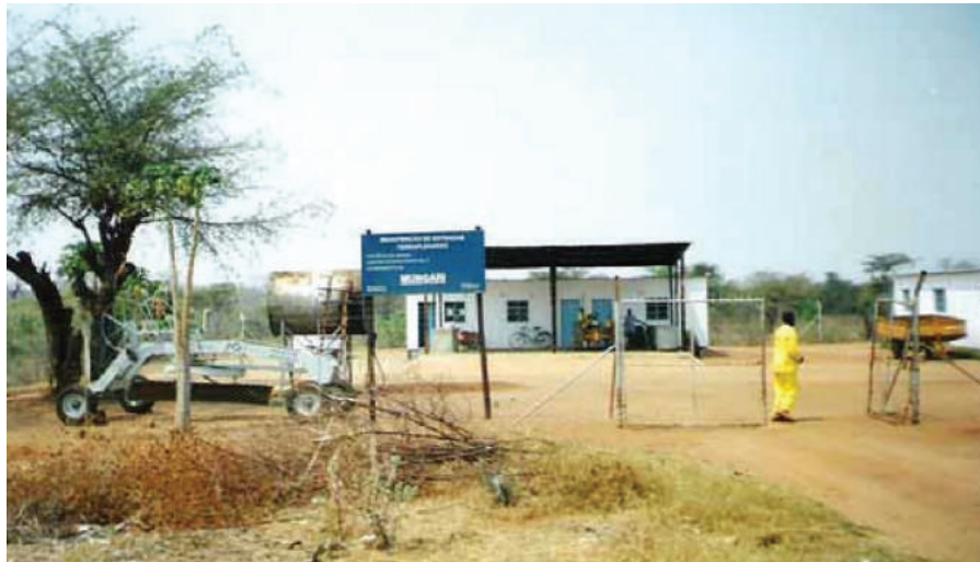
Figure E.4.1: Maintenance base camp in Zimbabwe
