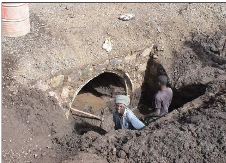
Figure E.7.2: Cleaning the drop inlet and barrel of a large bore culvert
