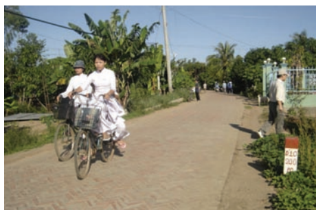
Completed brick paving road in service.
