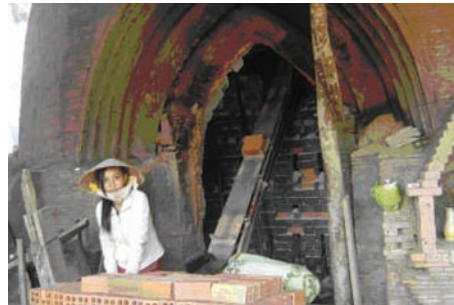
Unloading fired bricks through the kiln entrance with the aid of an electric powered conveyer. (Note that the hollow bricks shown are not suitable for road paving).
