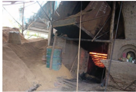
Husk feed hopper at kiln entrance. Firing in process.
