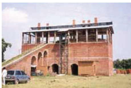
Vertical Shaft Kiln
