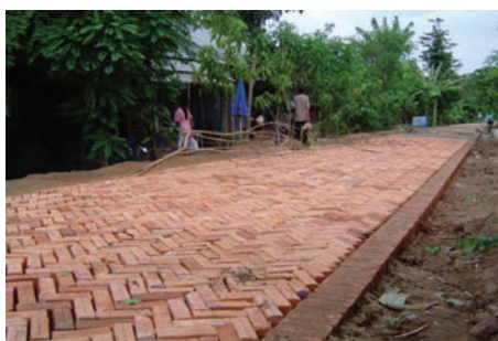
Brick paving laid and ready for sand-cement mortar jointing.
