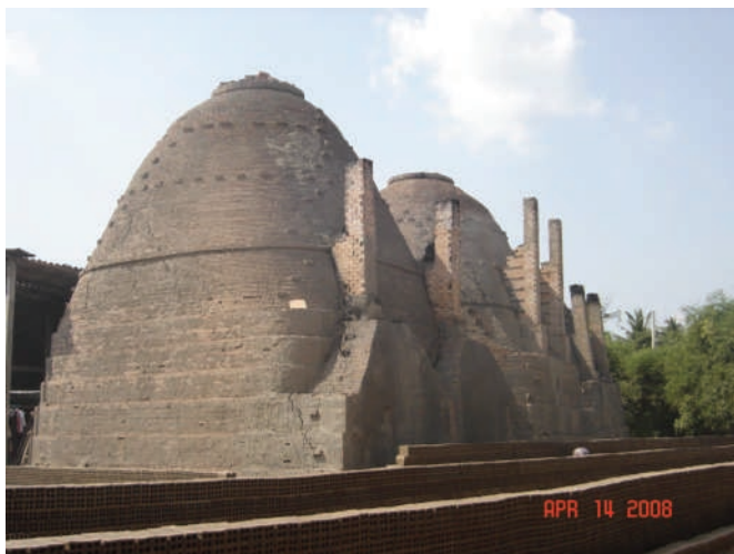
Figure 3 – Beehive or bell shaped kilns for rice husk firing of clay bricks
