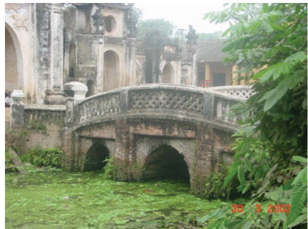
Figure 2 – Ancient Brick Bridge
