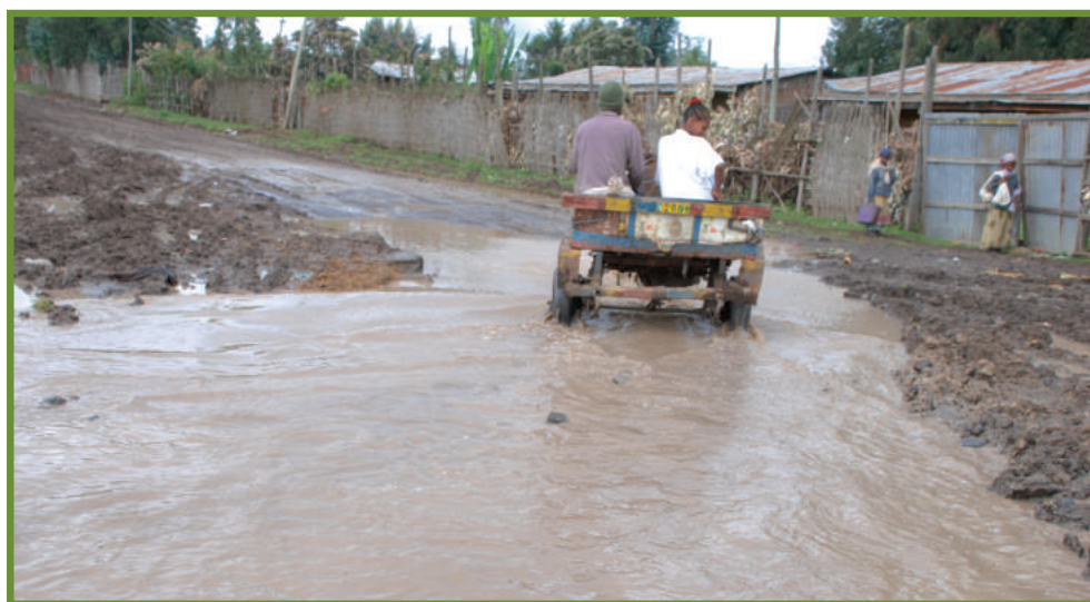
Plate A.1.1: Typical Access Problems
