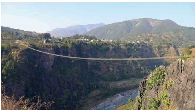
Figure 5: The Kusma Gyabi long span trail bridge
