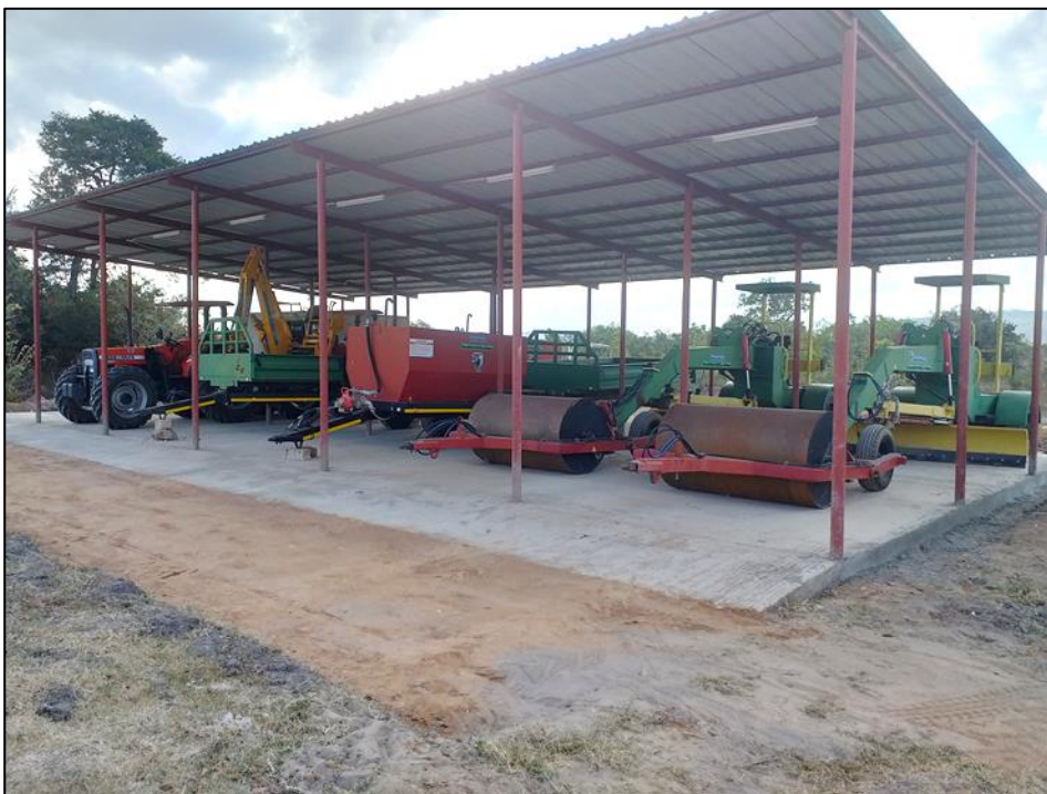
Figure 5 – Completed equipment shed at Kanakantapa Training Site
