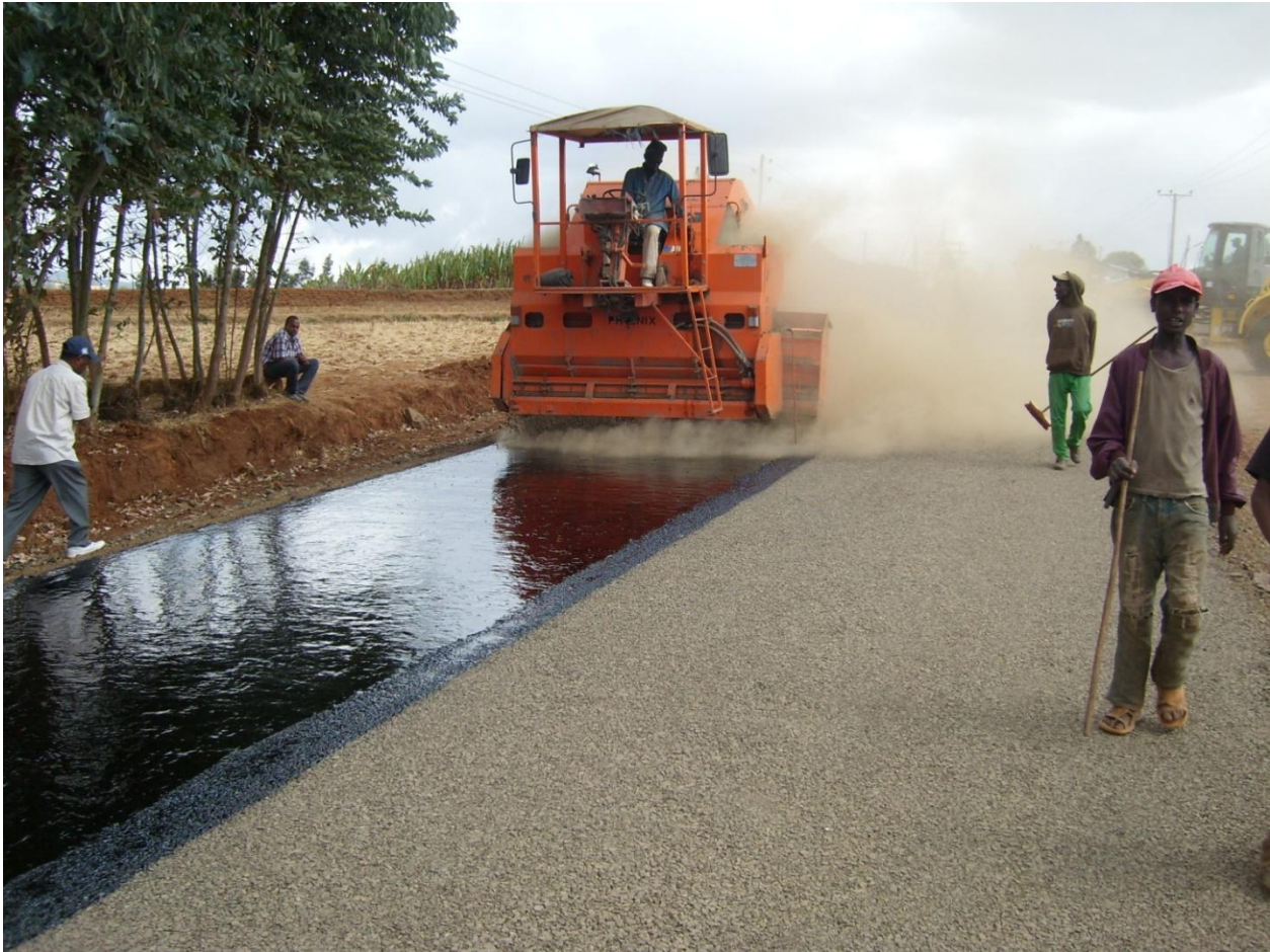
Figure 1 Construction of Otta Seal Demonstration Site in Ethiopia
