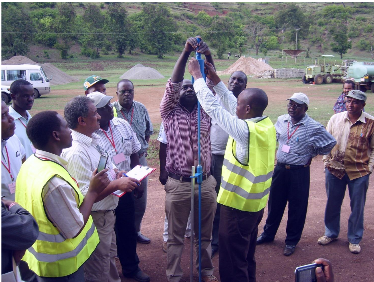
Figure 2 DCP Demonstration in Tanzania
