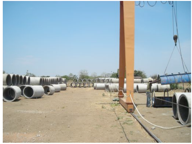
Plate 2 – Contractor's Camp in Katete – storage of 900mm Culverts
