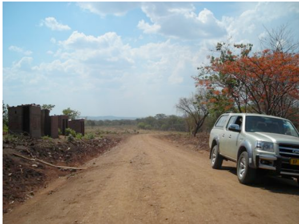
Plate 7 – RD687 – section due for full improvement (bush clearing and formation levelling has taken place
