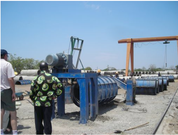
Plate 1 – Contractor's Camp in Katete – making of 900mm diameter culverts in progress
