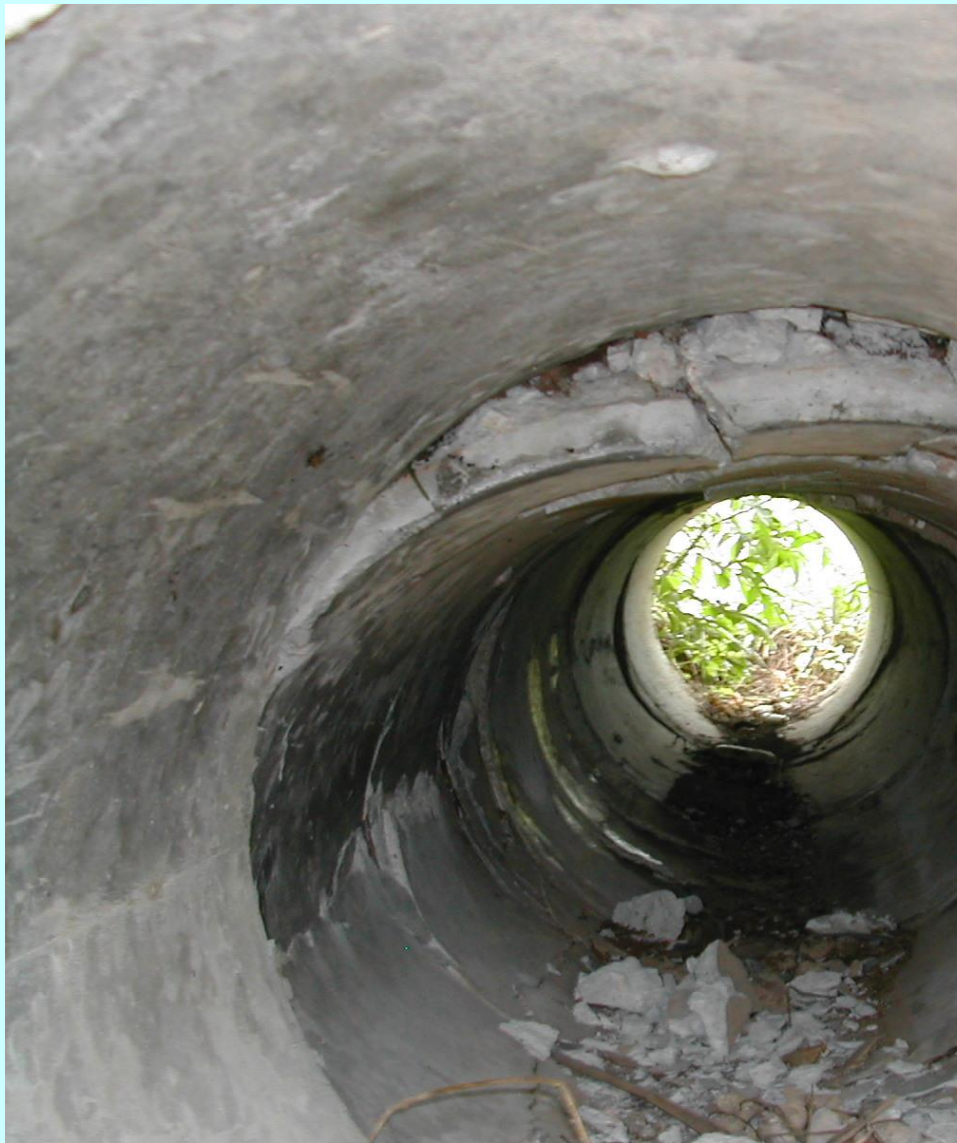
Rural Road Culvert damaged by Heavy Goods Traffic
