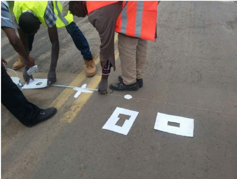
Figure 12: Across Africa team using the three road marking templates
