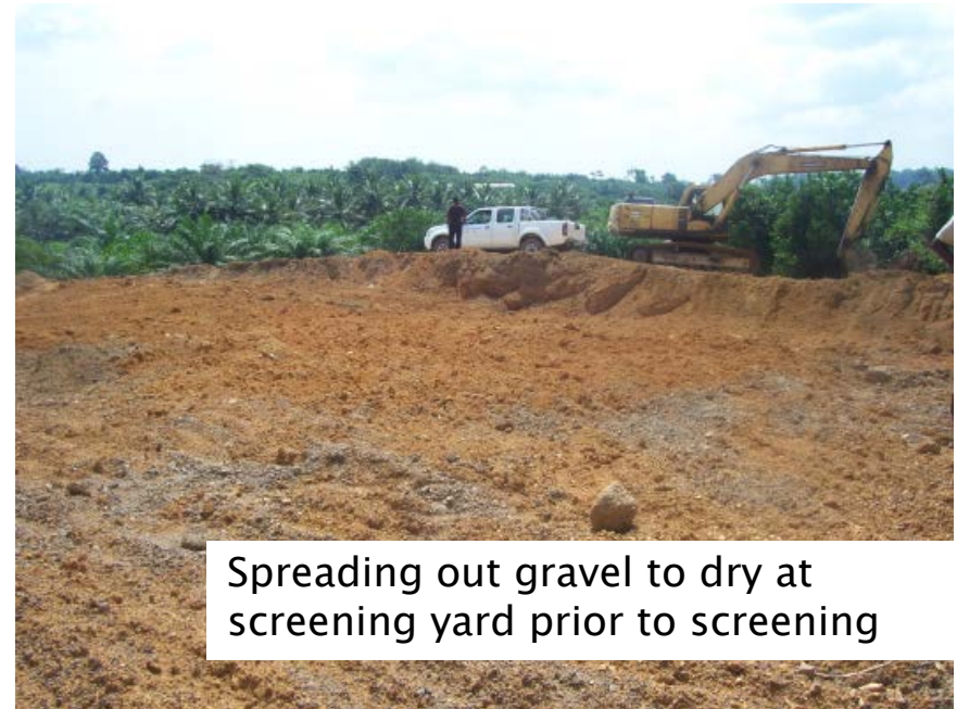
Excavating gravel from borrow pit to screening yard
