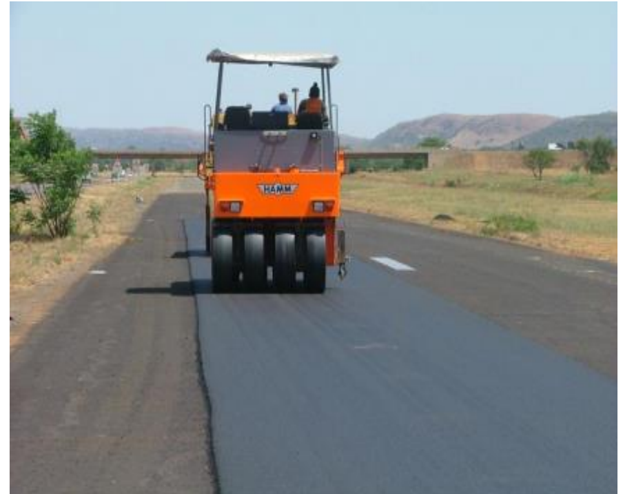
Thin hot mix asphalt
