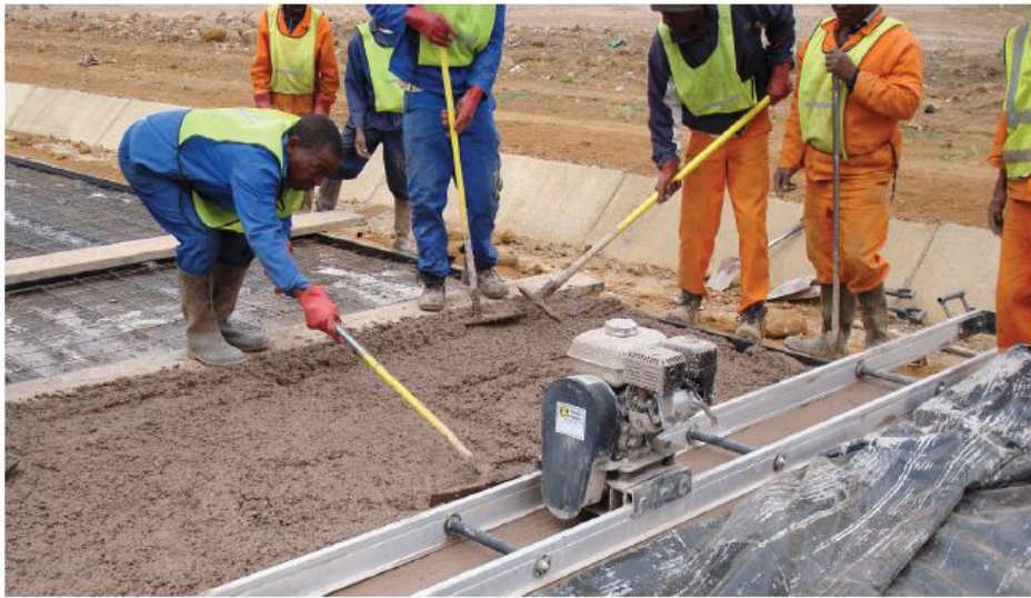
Labour-intensive construction of a low-volume road
