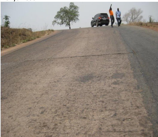
Reinforced Concrete Surfaced on 18% Gradient Section on Tafo-Nobi Road
