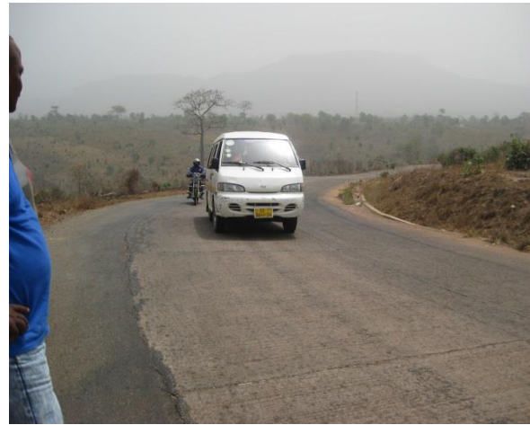
Sharp Curves on Concrete Section of Tafo-Nobi Road
