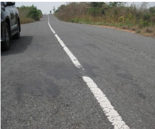
Patching of Bituminous Single Seal Surfaced on Aprade-Somanya Road
