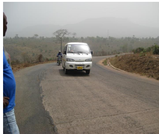
Rehabilitated Section with both Concrete and Bituminous Surfacing
