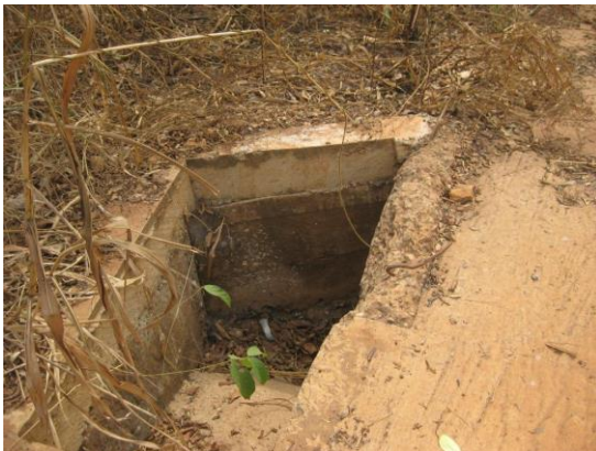
Drainage Structure on Concrete Surfacing Road Section
