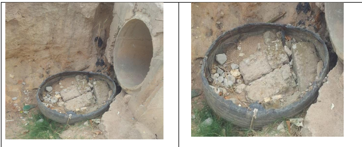
Figure 5-2: Photos showing innovative use of worn-out tyre (a waste material) for erosion check
