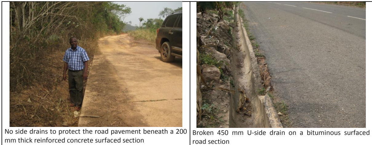
Figure 6-3: Different types or absence of road side drainage structures
