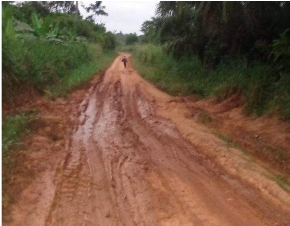
Figure 1: Road section requires proper drainage /surfacing intervention
