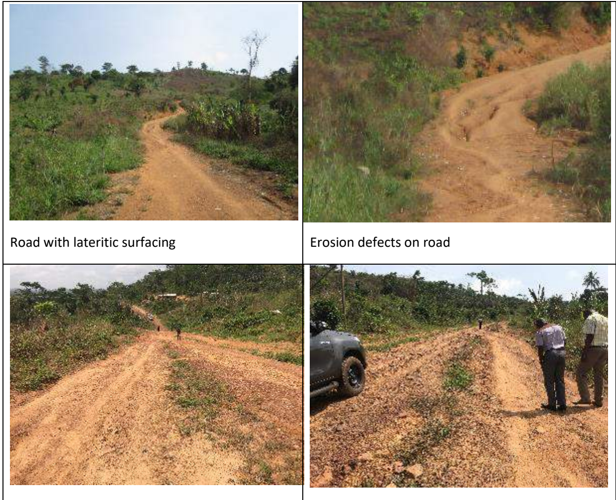
Figure 15: Some terrain features of KloAgogo– Oluhai road
