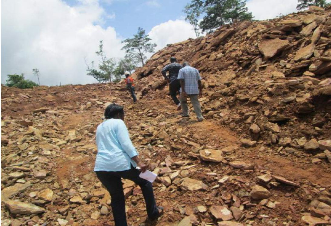
Figure 19: Road section on a slope ~ 20% with rock fragments
