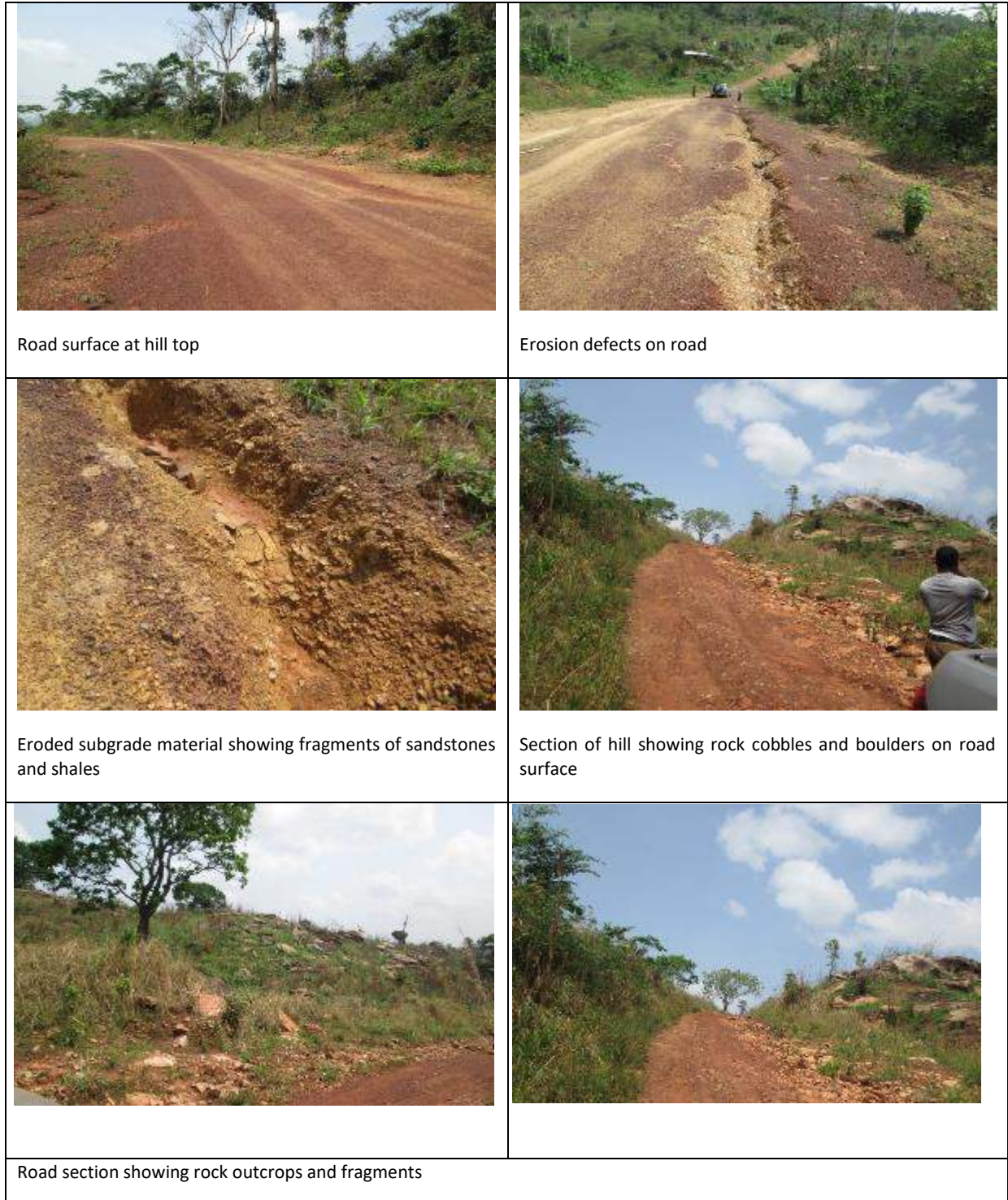
Figure 11: Some terrain features of Akatawiah – Terwanya road
