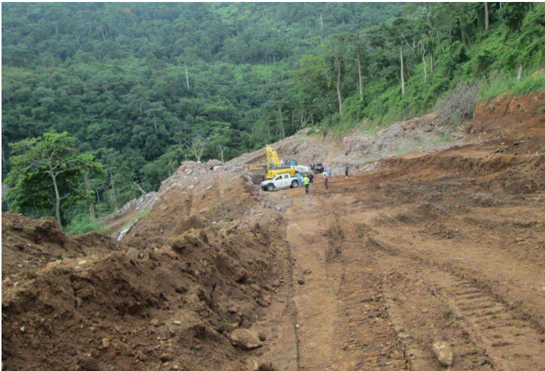
Figure 20: Road section on a slope ~ 20%, requires effective drainage systems
