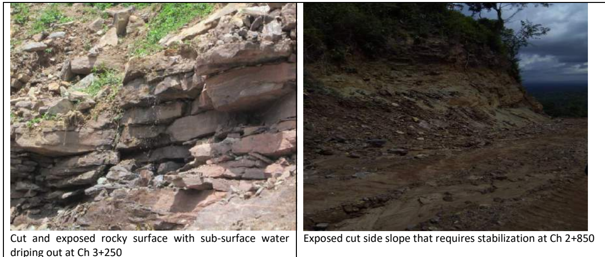
Figure 17: Some terrain features of Akwasiho - Twenedurase road
