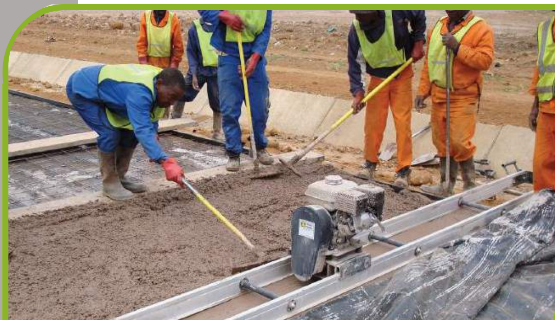
Labour-intensive construction of a low-volume road
