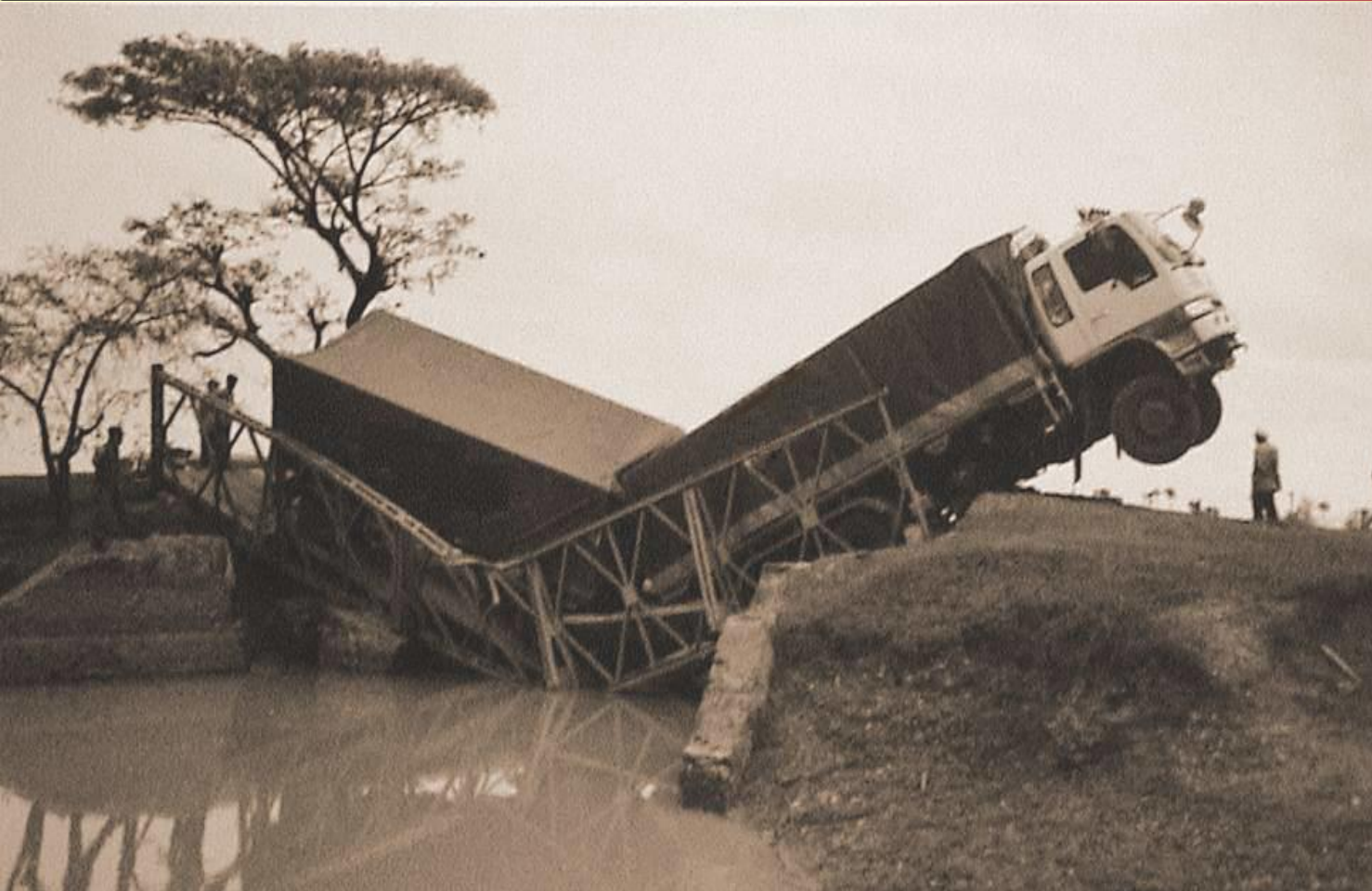
Collapsed Bridge along Secondary Roads
