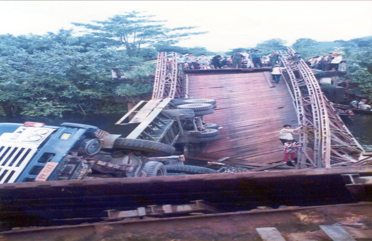
Collapsed Bridges on RN3
