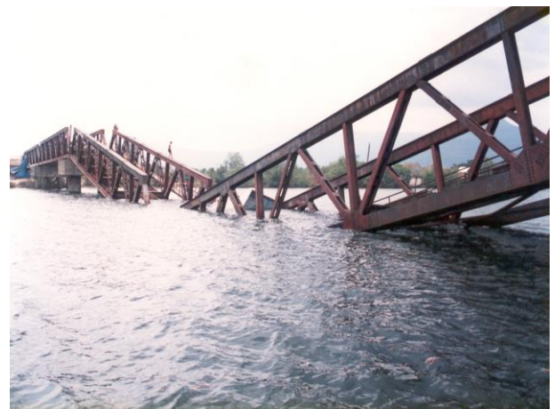
Collapsed Bridge on Rail Bridge
