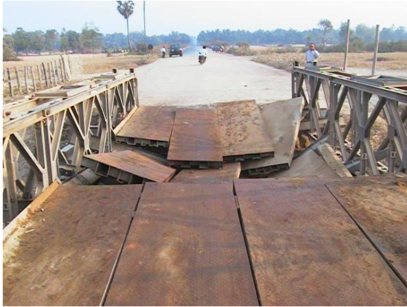
Collapsed Bridges on RN5
