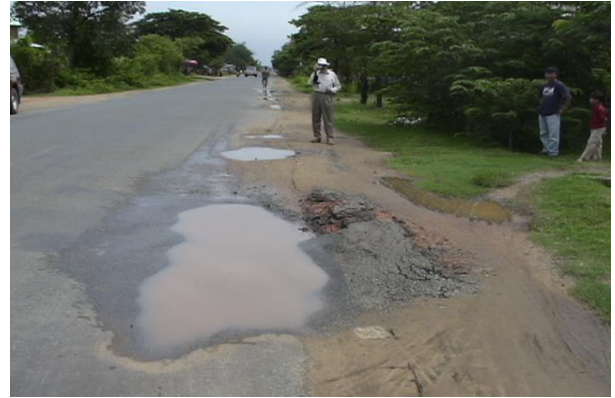
Damaged road pavement along Primary Road
