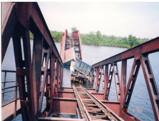
Collapsed Bridge on Rail Bridge
