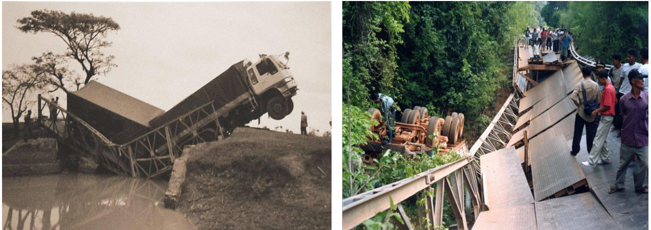
Collapse Bridge along Secondary Roads
