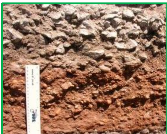
GCS base over natural gravel sub-base
