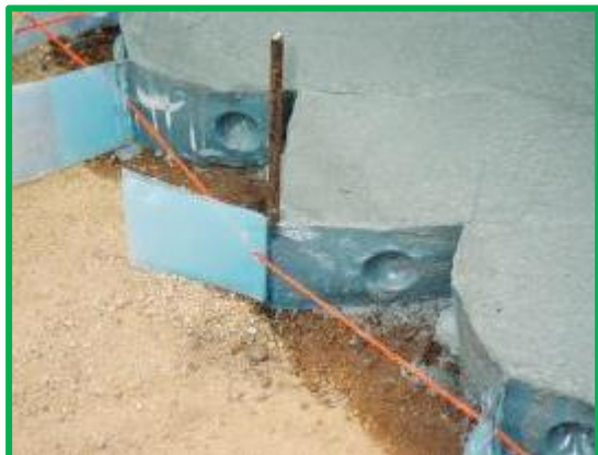
Geocells during construction
