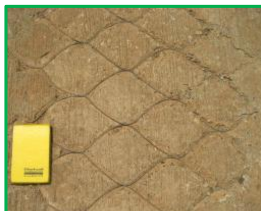
Geocell pavement 2 years after construction
