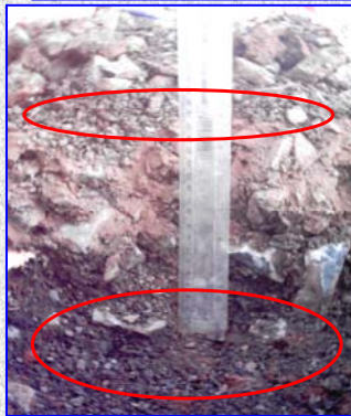
Poor grading and segregation in macadam
