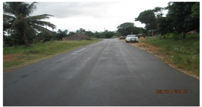
Fig. 6. Armured base sections on flat terrain.
