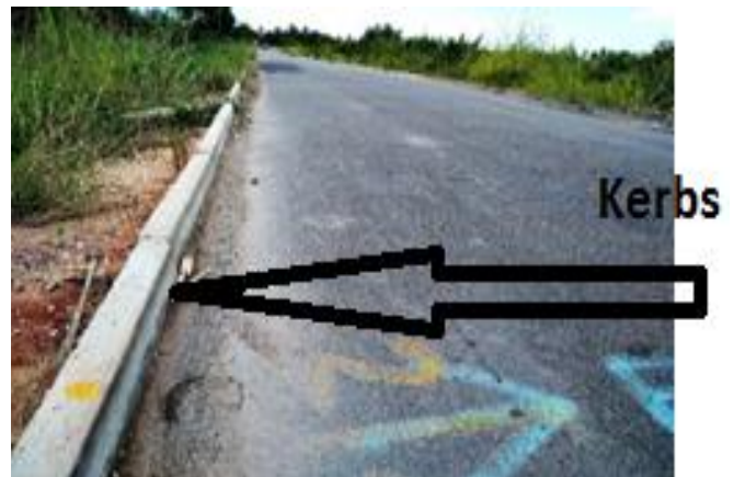
Fig. 8. Kerbs on blended base section
