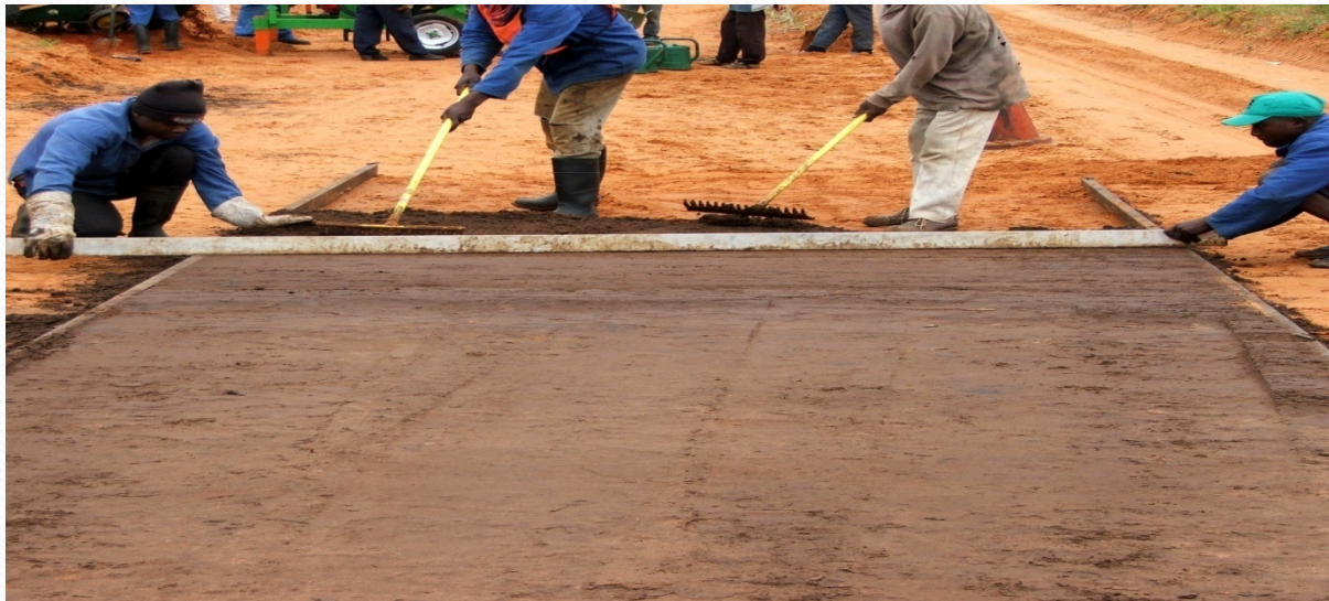
SPREADING MIXED S.T.E. NEXT TO TRANSVERSAL JOINT
