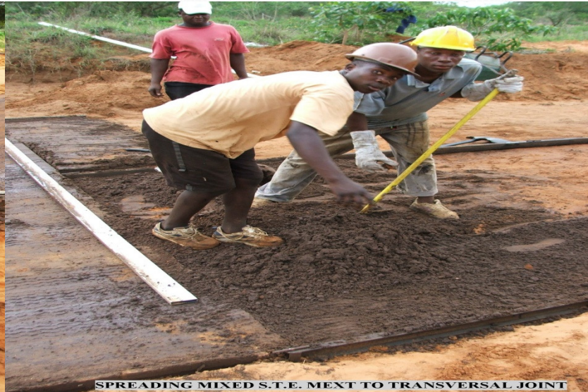
SPREADING MIXED S.T.E. NEXT TO TRANSVERSAL JOINT
