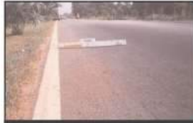
Low severity with rut depths < 12 mm
