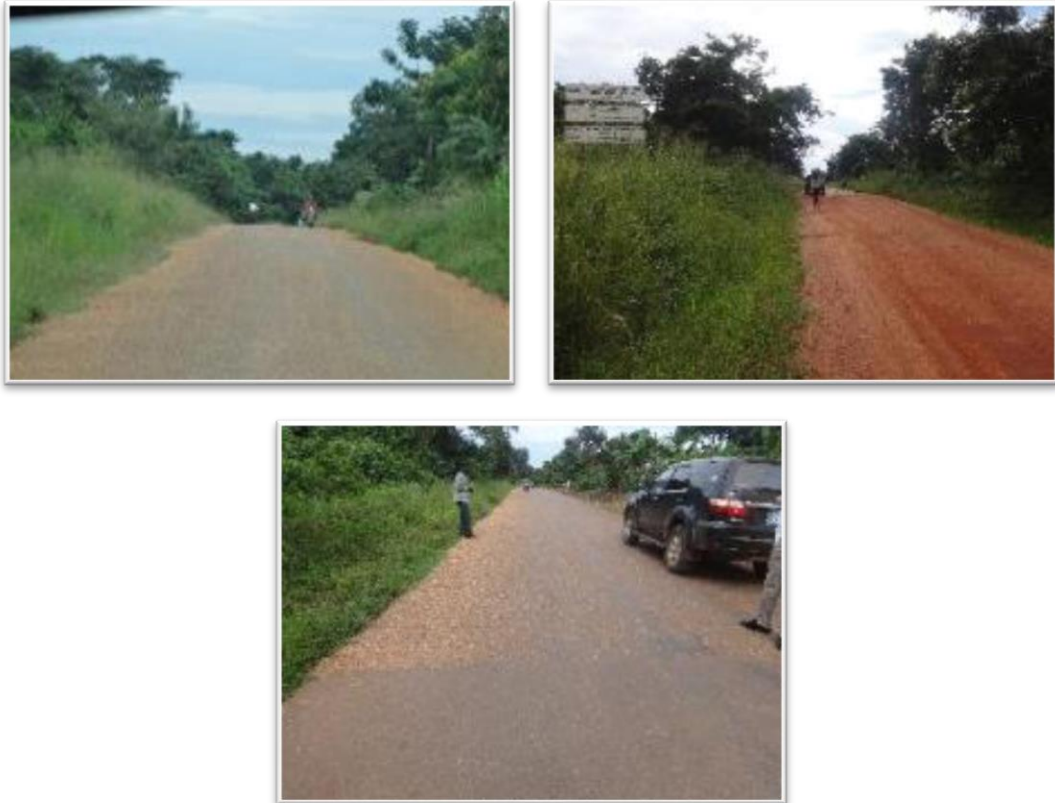
Figure 10: Uganda Site Visit Kasiso-Logwi Road
