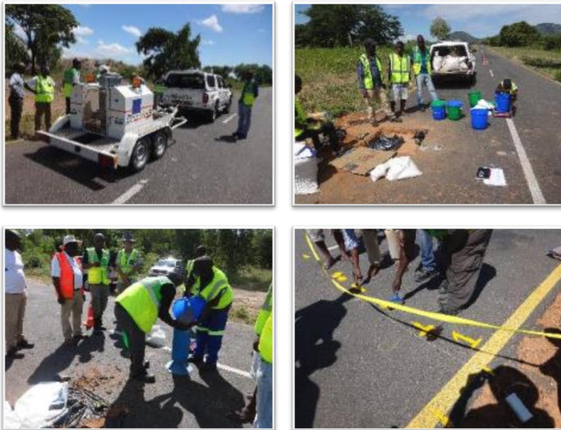
Figure 1: Site work on T357 Parachute Battalion – Lifuwu Road
