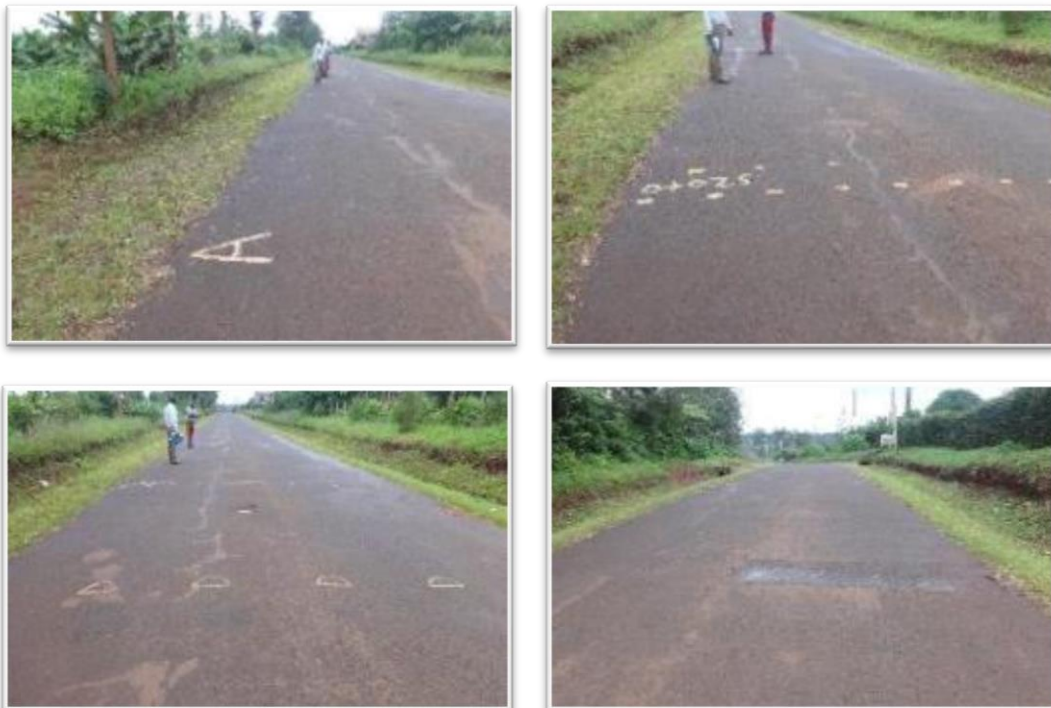
Figure 8: Wamwagi Karatu Road Monitoring Section
