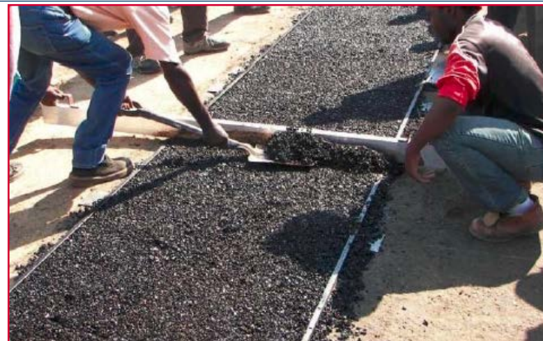
Thin cold mix asphalt
