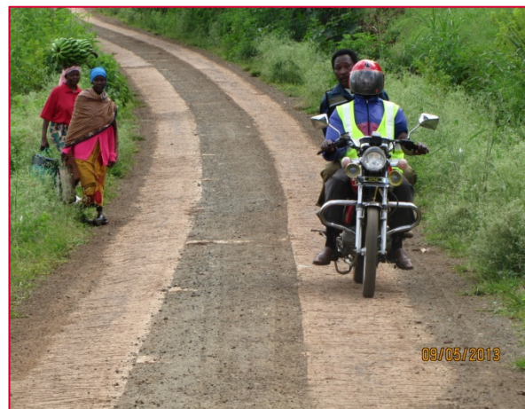
Concrete slabs and block paving
