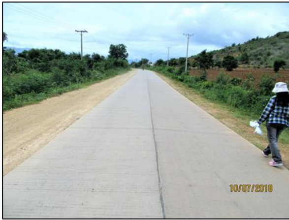
Unreinforced Concrete Slabs
