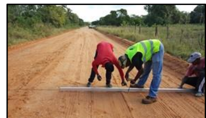
Control Section after grader blading
