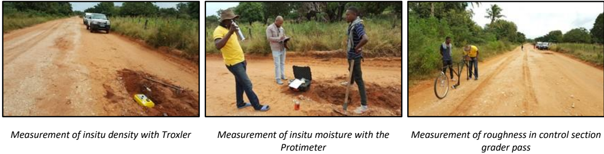
Figure 2.7: Team work on Gravel Control Section
