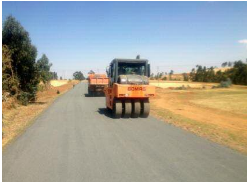
Figure 5-2 A completed section of the Combel trial
