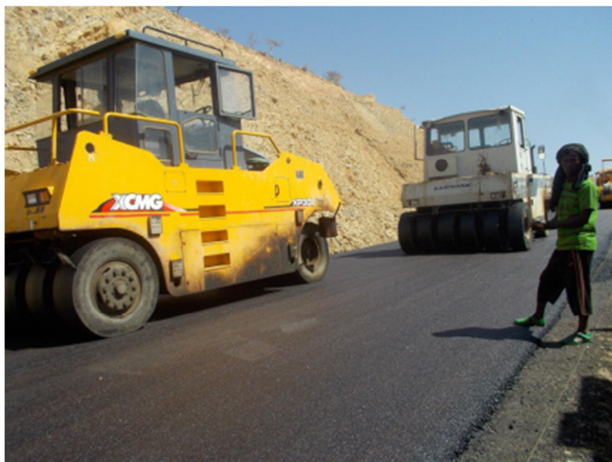
Figure 7-4 Compaction of the asphalt surfacing
