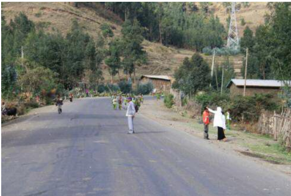
Figure 6-4 Completed Otta seal surfacing near the school
