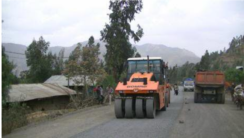
Figure 6-2 Rolling with pneumatic roller and tipper truck
