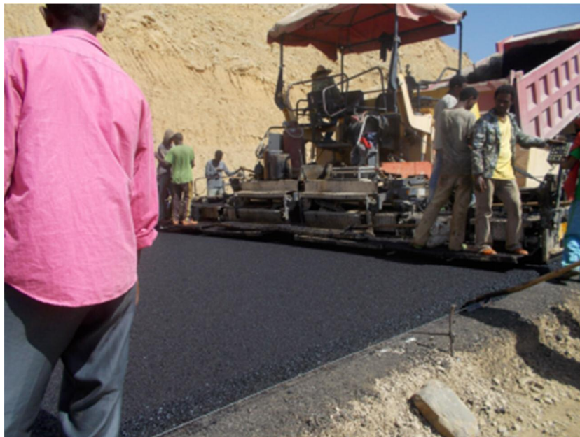
Figure 7-3 Laying of the asphalt layer by paver
