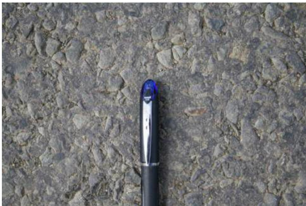
Figure 6-3 Close-up of the broomed surfacing applying the 2 nd seal
