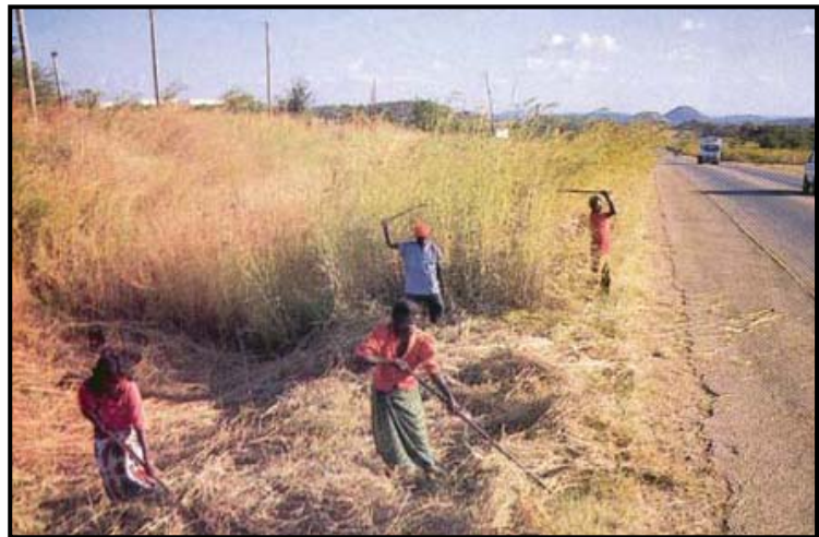
Photo 1: Grass cutting – a typical labour-based routine maintenance activity.
