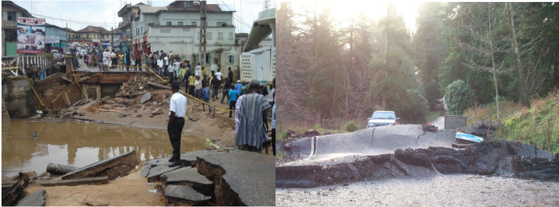
Extreme climate events are causing damage to infrastructure
