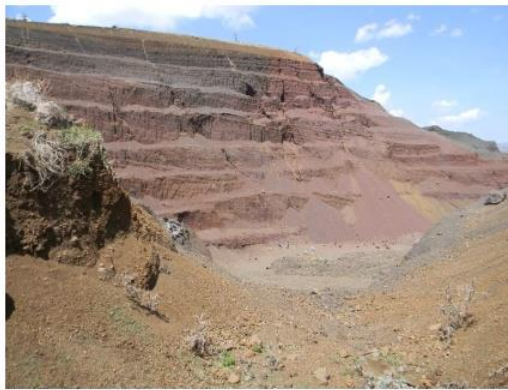
Benched excavation into consistently-dipping scoria
