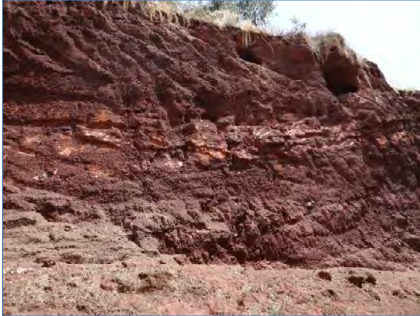
Figure 12: Side of the borrow pit worked by dozer
