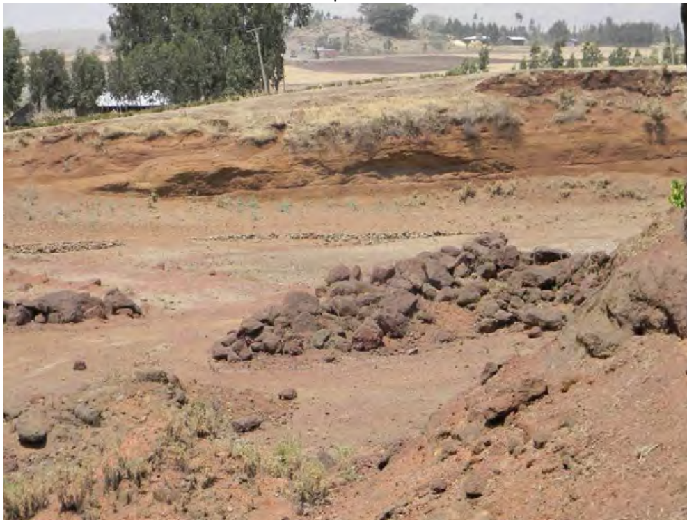
View approx. west, looking down-dip at Material 3 in the far excavation with boulders of Material 1 in the middle ground
