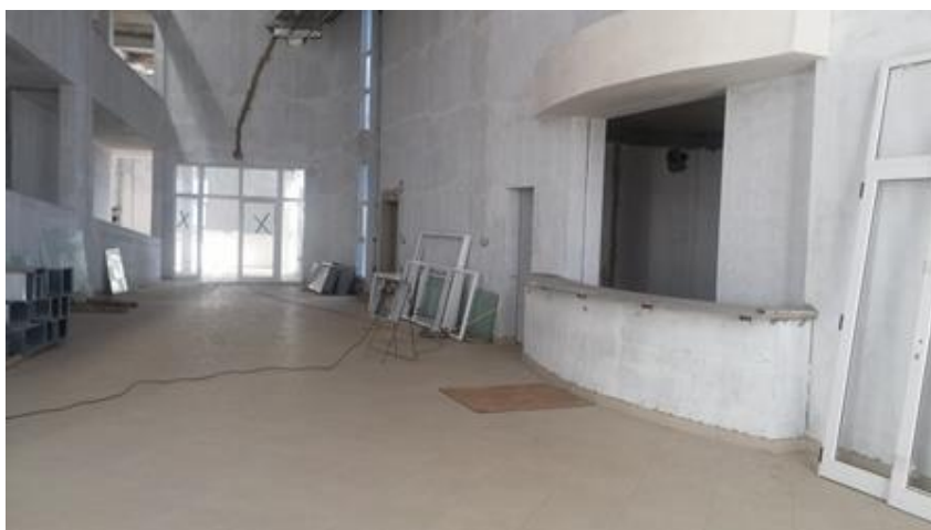
Figure 2: Auditorium foyer (under construction)
