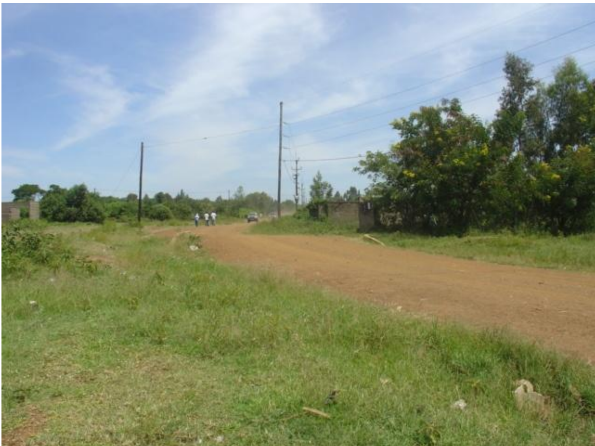
Picture 2: Example of hump constructed over a culvert to avoid lowering the invert. Drifts would probably be a better solution in this type of terrain.
