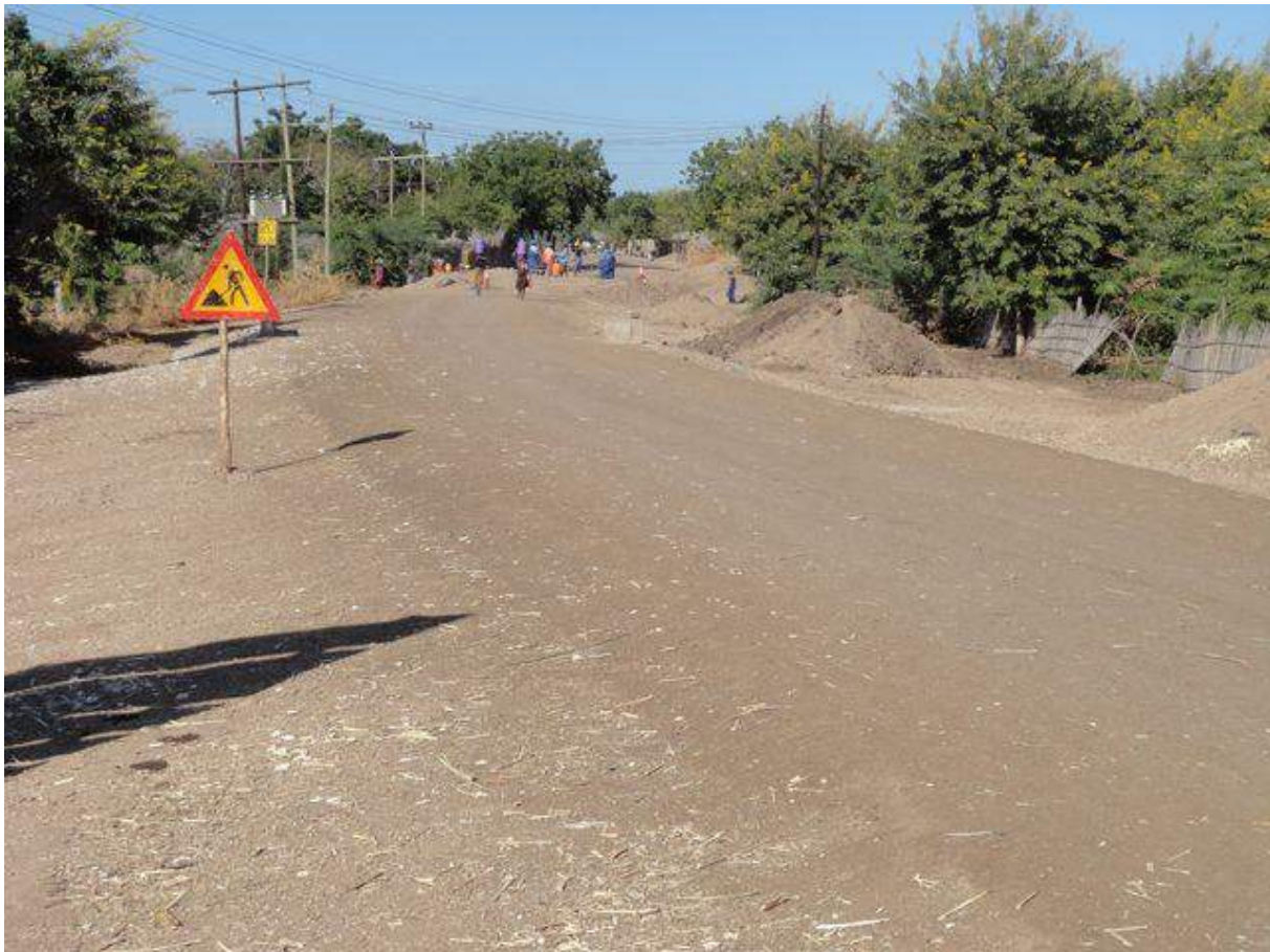
Figure 2: Start of D387 at junction with M1
