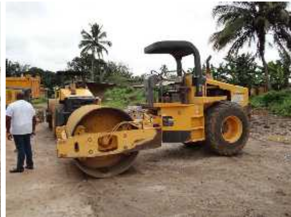
Figure 3: One of the two 10-ton vibrating rollers
