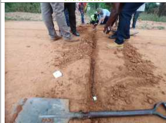
Figure 23: Installation of sensors in the base
