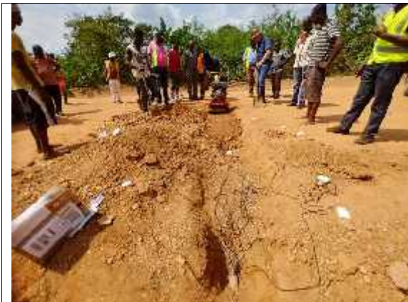
Figure 21: Installation of sensors in the subgrade and subbase
