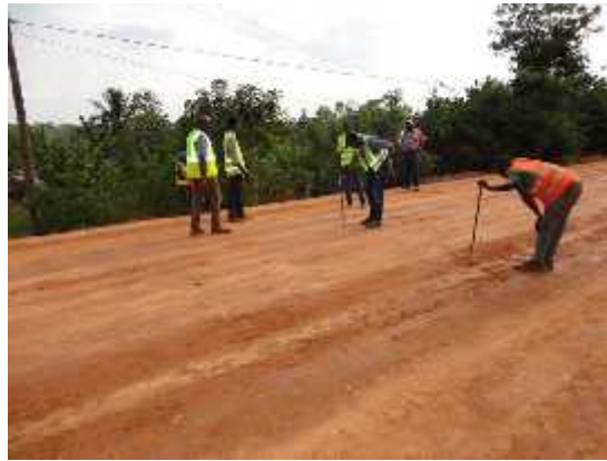
Figure 11: Checking the camber
