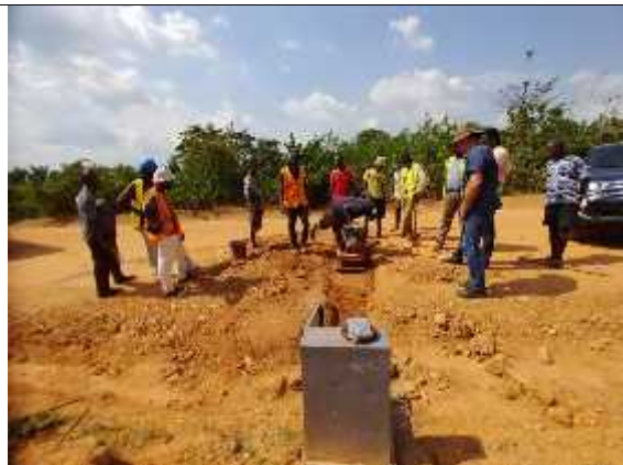
Figure 22: Compaction of trench after installation
