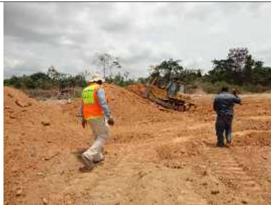
Figure 6: Stockpiling in process
