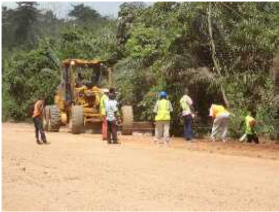
Figure 10: Establishing level pegs
