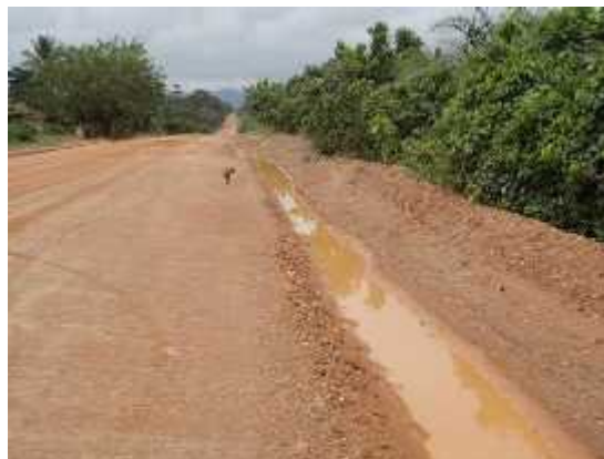
Figure 13: Windrows on backslope to be removed
