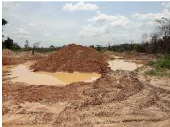
Figure 7: Flooding of the borrow pit
