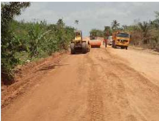
Figure 12: Correcting the camber to +/- 3%
